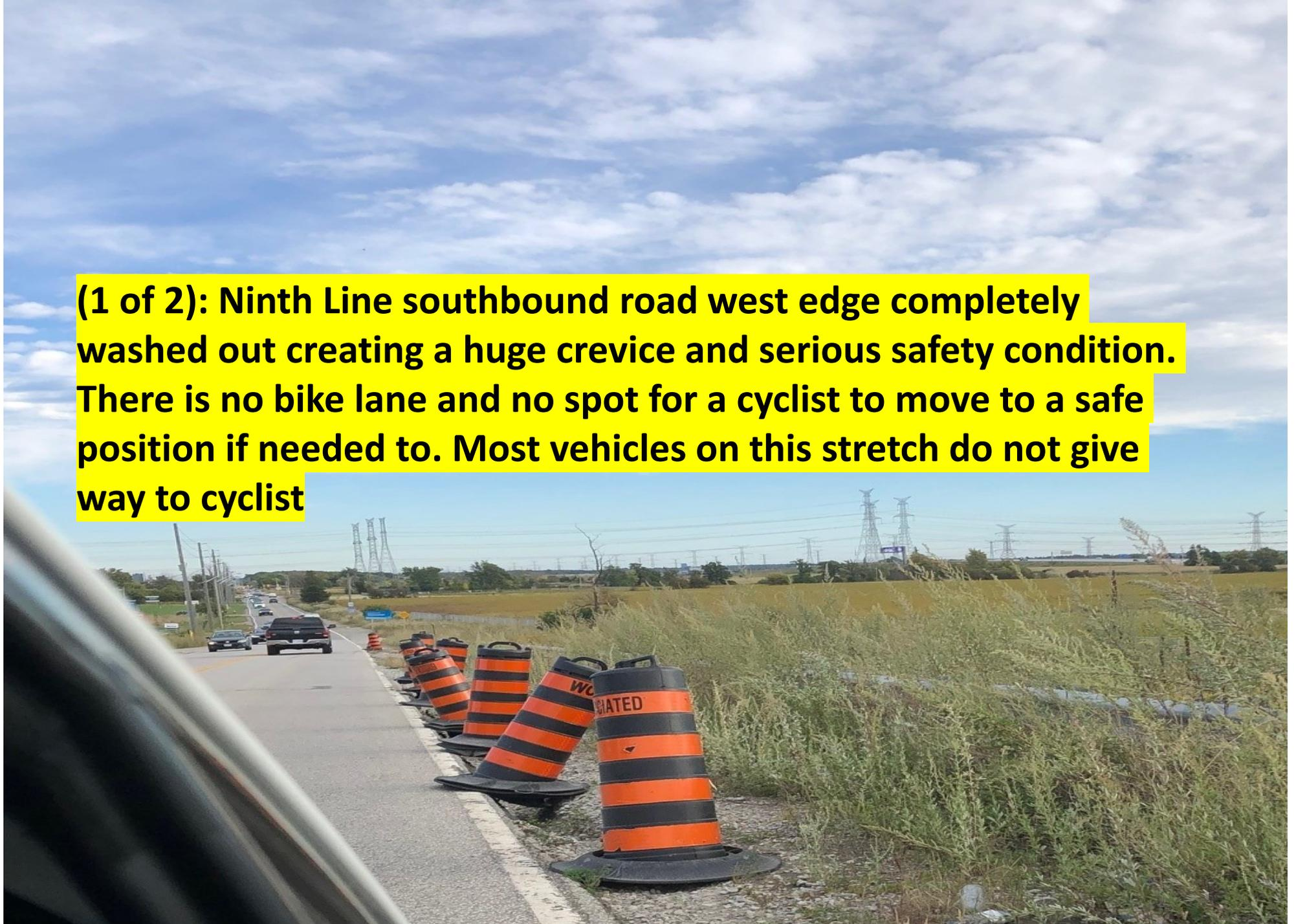
**(2 of 2): Ninth Line southbound road west edge completely washed out creating a huge crevice and serious safety condition. There is no bike lane and no spot for a cyclist to move to a safe position if needed to. Most vehicles on this stretch do not give way to cyclist**
