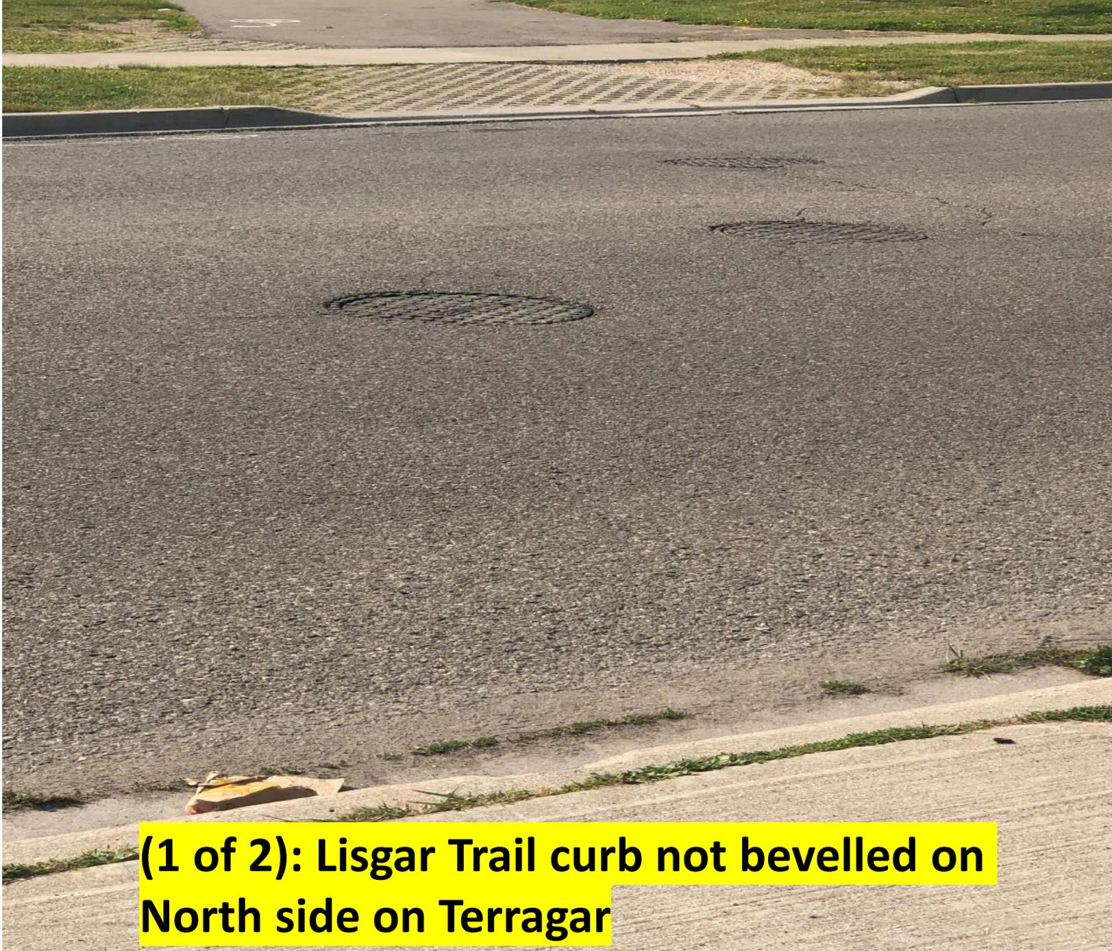
**(1 of 2): Lisgar Trail curb not bevelled on North side on Terragar**
