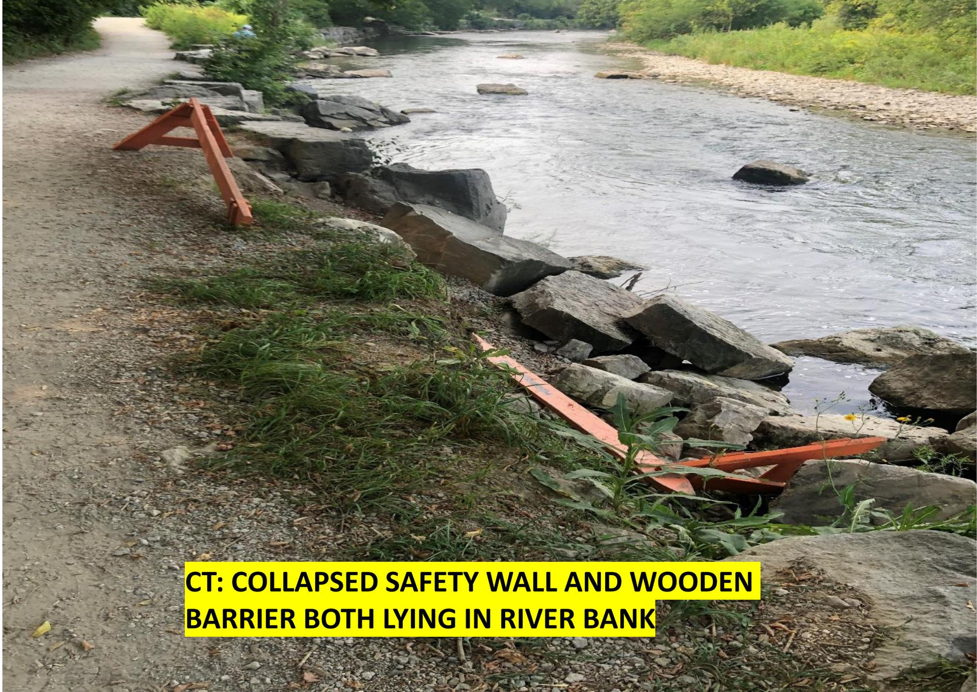
**CT: COLLAPSED SAFETY WALL AND WOODEN BARRIER BOTH LYING IN RIVER BANK**
