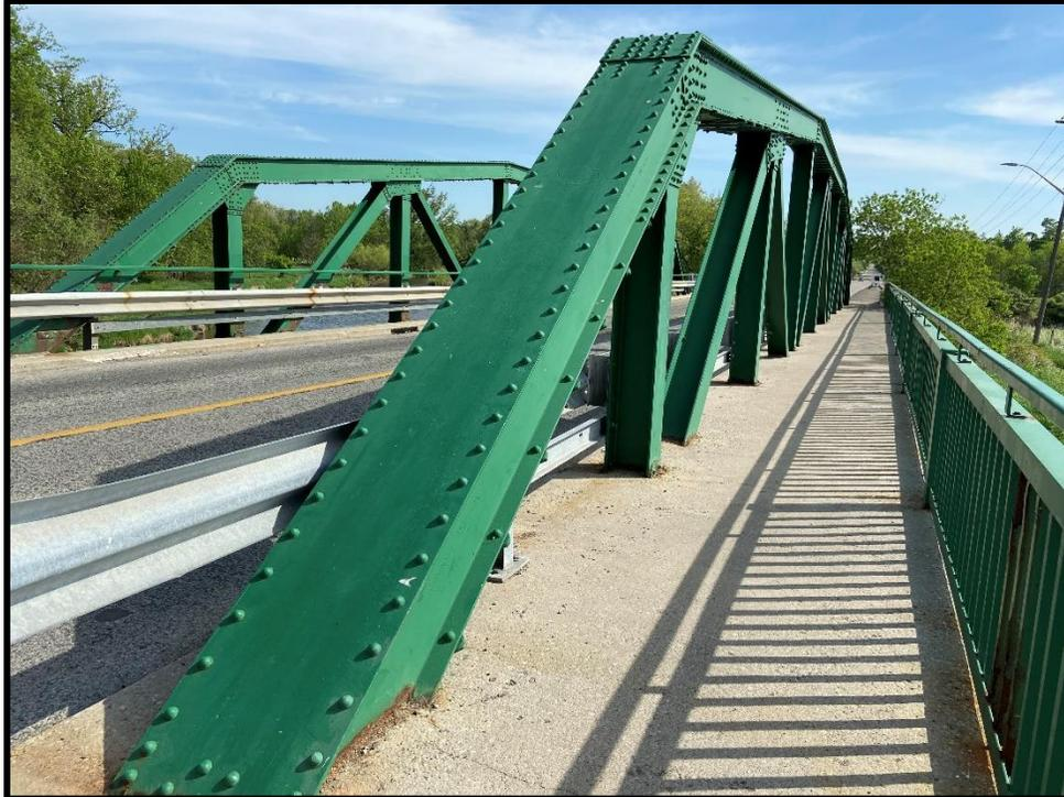
**Image 17: Detail of End Post, South Truss and Sidewalk
