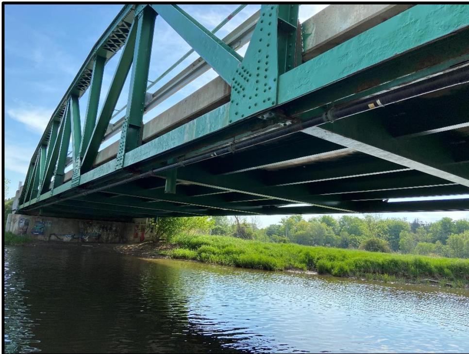
**Image 28: Detail of Floor Beams and Stringers, Underside of Old Derry Road Bridge
