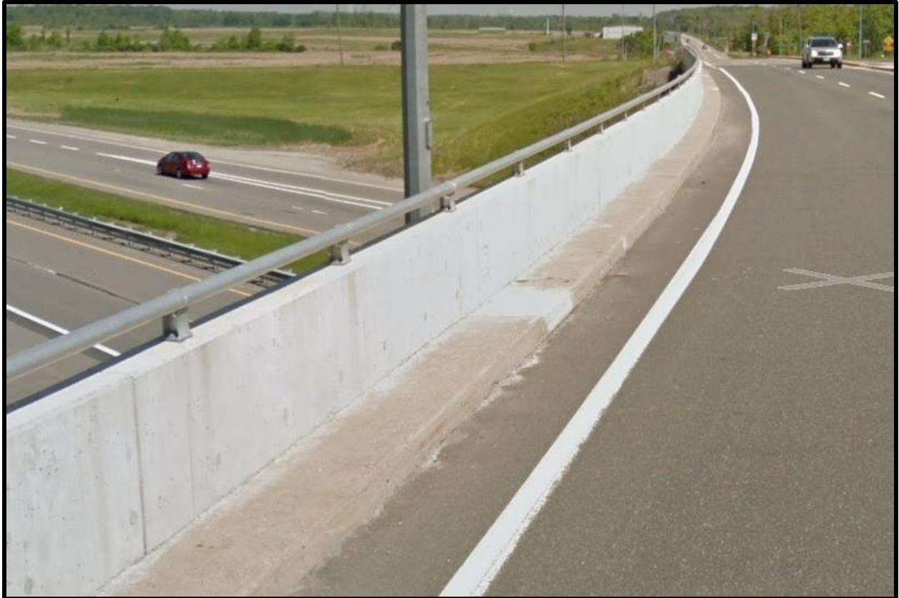
**Figure 8: Example of Guardrail Option 1: Concrete Parapet Wall**
