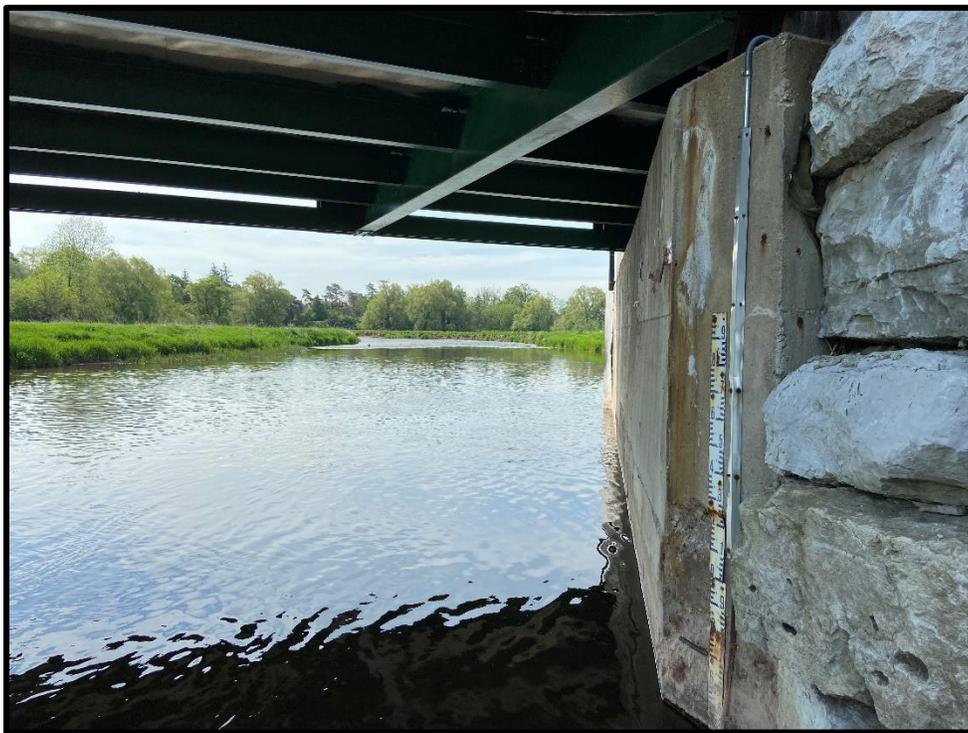
**Image 26: Detail of Old Derry Road Bridge Stringers and West Abutment**
