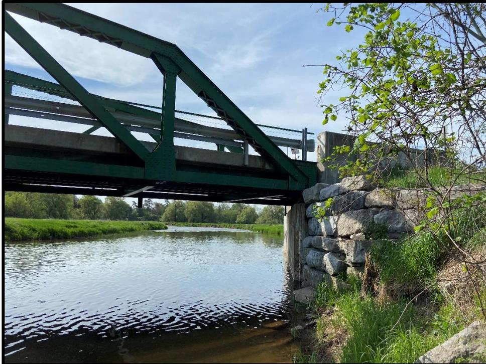
**Image 25: Detail of Masonry Gravity Retaining Wall, Northwest Side of Old Derry Road Bridge**
