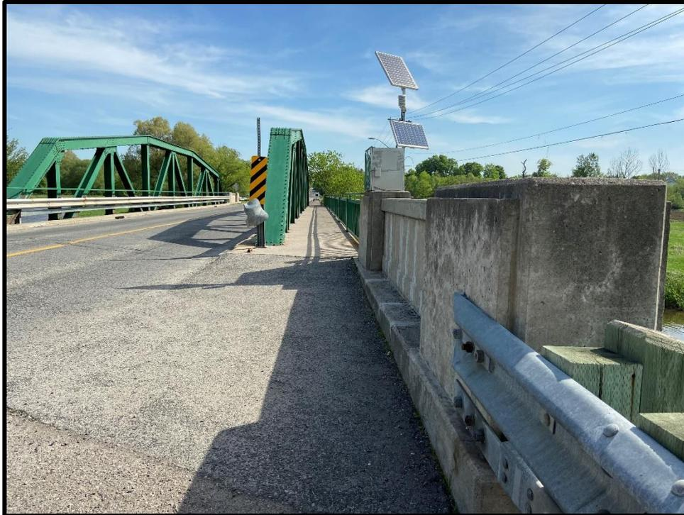
**Image 15: Detail of Old Derry Road Bridge South Sidewalk and Barrier Wall
