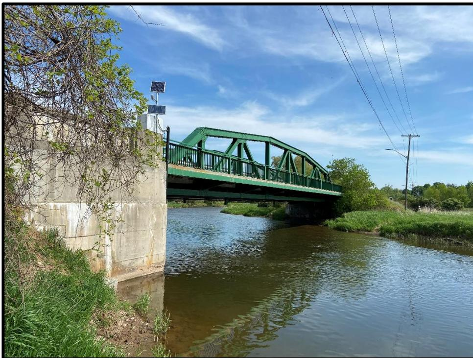
**Image 12: Old Derry Road Bridge West Abutment and South Wing Wall
