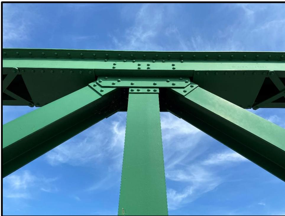
**Image 20: Detail of Top Chord Connection, South Side of Old Derry Road Bridge
