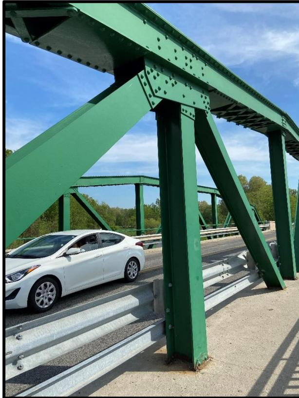
**Image 19: Detail of Diagonal and Vertical Members and Rivets, South Side
