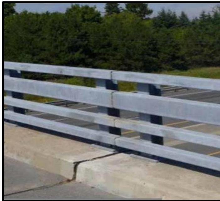
**Figure 9: Example of Guardrail Option 2: 4-Tube railing Steel Barrier**
