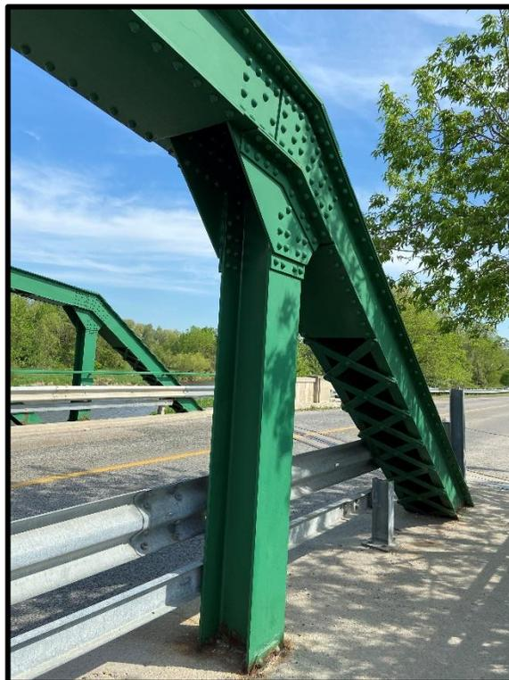
**Image 8: End Post Detail, South Side of Old Derry Road Bridge
