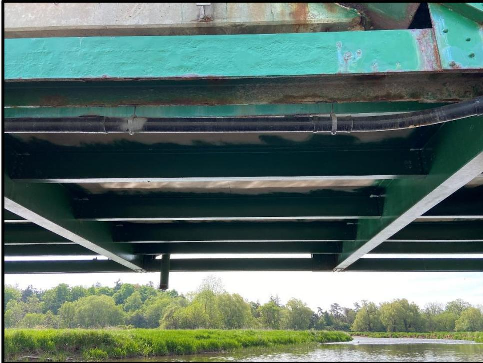
**Image 29: Underside Detail of Stringers, Old Derry Road Bridge
