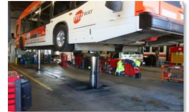
Transit Terminal Hoist Renewal
