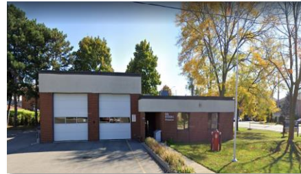
Fire Station Renovation Program
