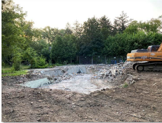
2515 Shepard Ave – Demolished
