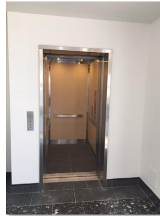
New LULA Elevator - MiWay Administration Centre
