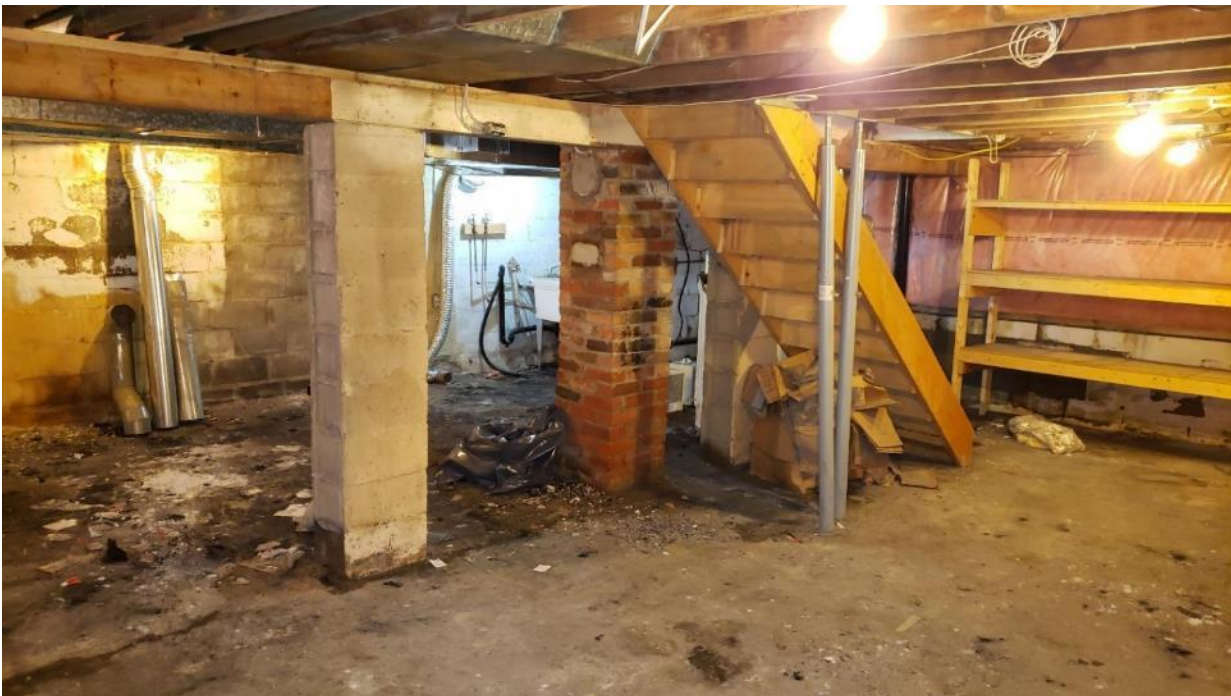
Figure 20 The basement of 40 Peter Street South showing added bracing for the main floor. ( Photo from client. )
