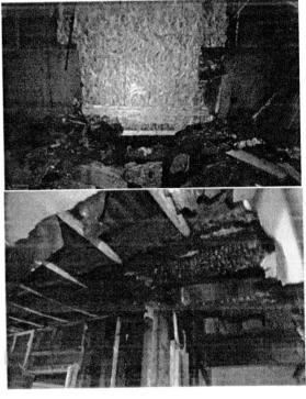
3. Smoke propagation has extended into the first floor masonry walls which are compromised and will be difficult to seal. These will also require replacement complete.
