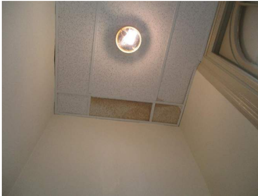
Photo # 23: View of stained ceiling tile in the women's washroom (north elevation, west addition).
