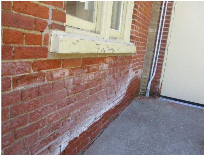
Photo # 10: White staining (efflorescence) was observed to be concentrated approximately 12 inches above grade level at the north and east elevations (original building).
