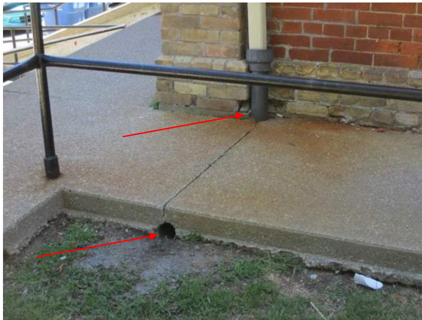
Photo # 14: A rain water leader was observed to be present next to the north-east corner pilaster at the north elevation and appeared to run underneath the access ramp.
