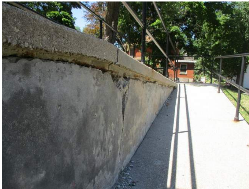
Photo # 21: View of typical deterioration at the access ramp on the northeast elevations of the building adjacent the northeast pilaster (original building and south addition, facing north).
