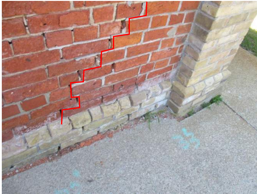
Photo # 13: View of step crack continuing through masonry brick at east elevation and mortar deterioration.
