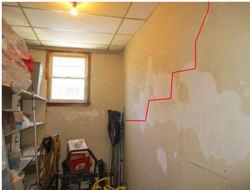
Photo # 24: Paint peeling was observed in jail cell 1 at the west elevation and a step crack was observed on the interior wall in between jail cells 1 and 2
