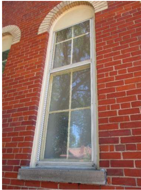
Photo # 19: View of typical single hung wood framed window with masonry arches and exterior aluminum framed storm windows at the exterior (south elevation of west addition).
