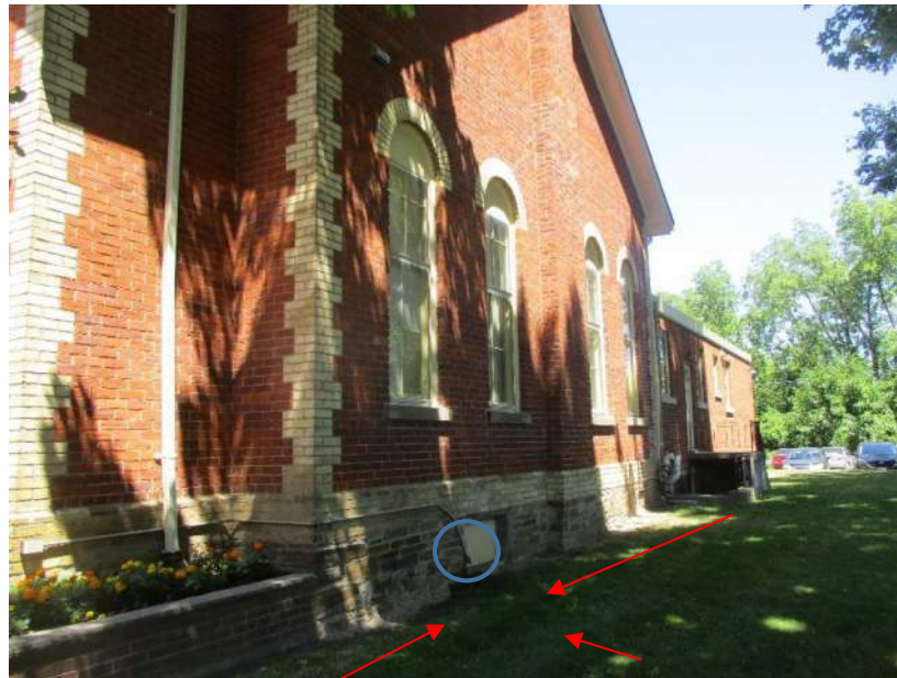
Photo # 17: View of a potential negative drainage at the west end of the south elevation. The direction of the approximate ground slope is shown with a red arrow, and the location of a leaking water tap is shown in blue.
