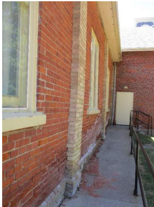
Photo # 7: Overview of spalling brick and efflorescence at the north elevation (original building, facing west).
