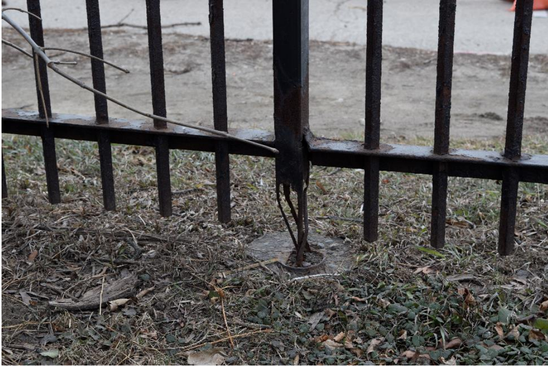
Image 15: Example of decay observed in the support posts of the fence.
