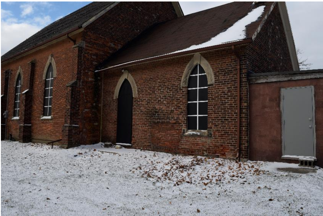
Image 10: Southeast side of Britannia United Church, note the missing mortar, mismatched bricks and grey spot repairs.
