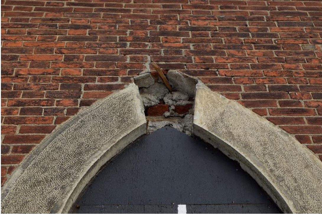
Image 11: Recent loss of key stone on north window of main façade.
