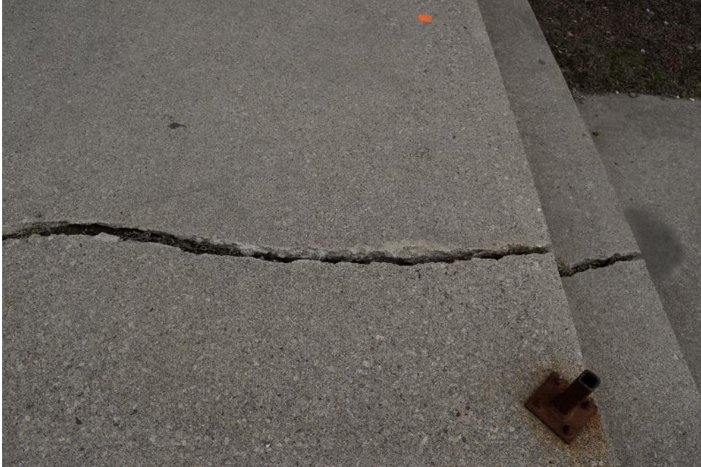
Image 5: Split in concrete, running full width of steps, note rusted mounting bracket for missing handrail.
