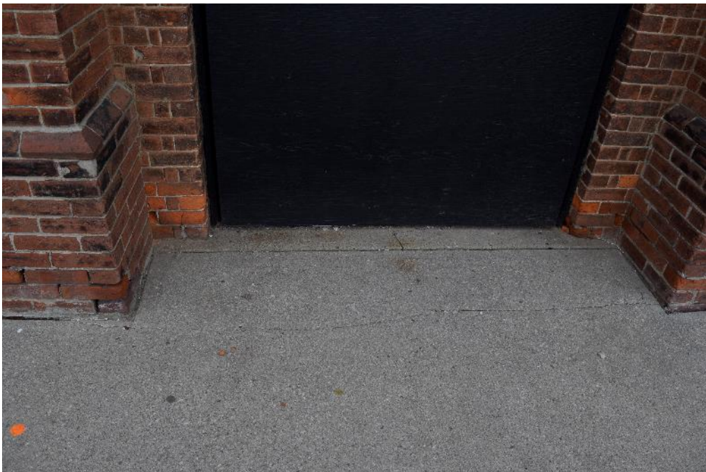
Image 6: Separation between concrete steps, landing and fabric of church.
