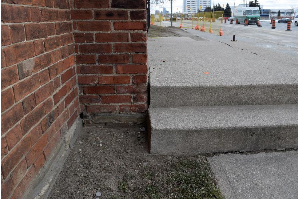
Image 7: Clear separation between concrete and fabric of church
