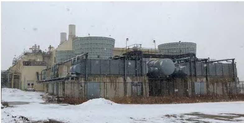
Co-generation plant, east and north elevations (ERA, 2020).
