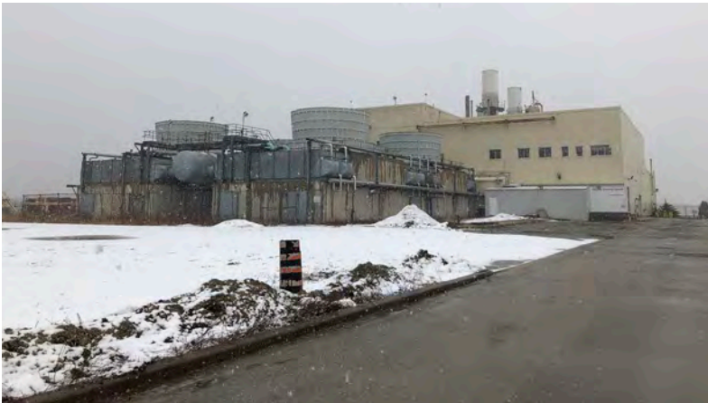
North elevation of co-generation plant (ERA, 2020).
