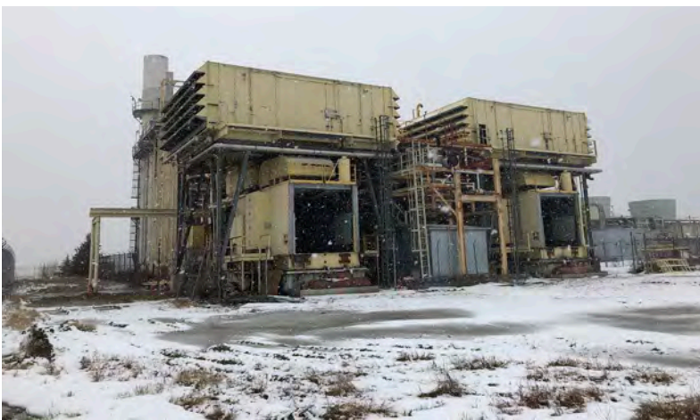
Co-generation plant, east elevation (ERA, 2020).
