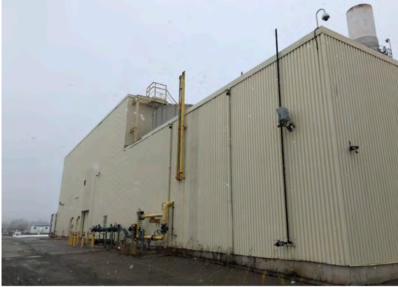
Co-generation plant, west elevation (ERA, 2020).
