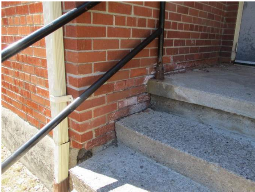
Photo # 6: Typical Masonry Brick and mortar deterioration at the eastern staircase.
