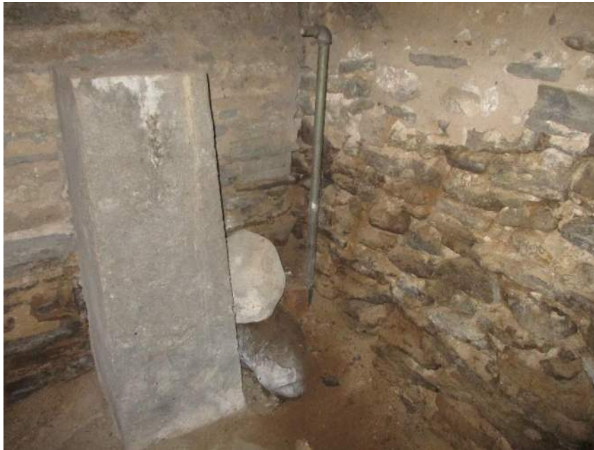
Photo # 27: View of typical deteriorated/lost limestone mortar at the base of the rubble wall foundation.
