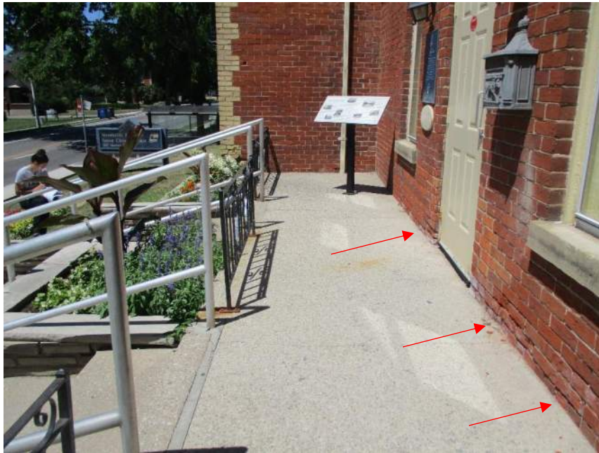
Photo # 9: View of mortar deterioration at the grade level of the west elevation (west addition).
