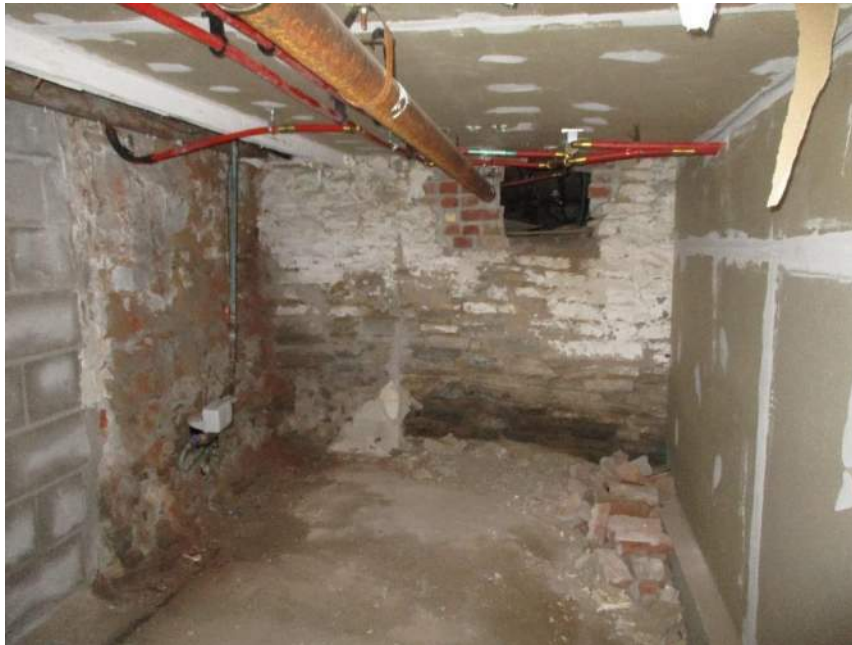
Photo # 25: View of rubble wall foundation. Moisture infiltration is visible at the base of the wall (north elevation, west addition).
