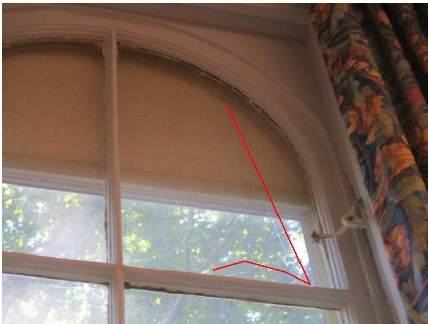
Photo # 20: View of crack in glass pane at wood framed window (south elevation, west addition).
