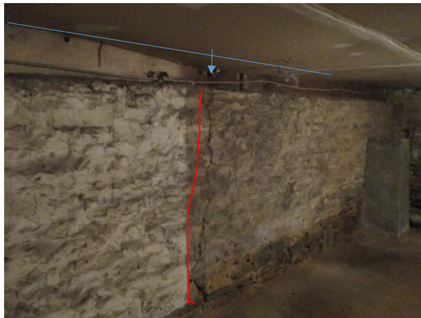
Photo # 28: The floor in the south kitchenette was observed to be bowing. View from below is shown with displacement in blue. A vertical crack in the rubble foundation wall below the bowed floor is shown in red.
