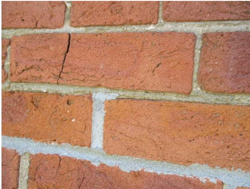
Photo # 11: View of the brick masonry at the east elevation. The masonry was observed to have a rough texture that appeared to be the result of sandblasting (original building).
