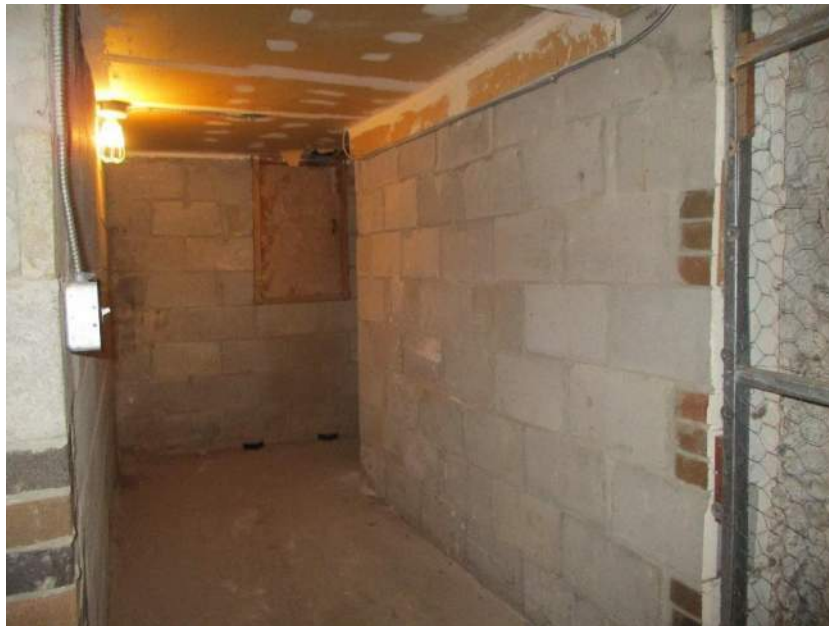
Photo # 26: View of typical concrete masonry unit foundation in the newer addition to the building (interior hallway, south addition).
