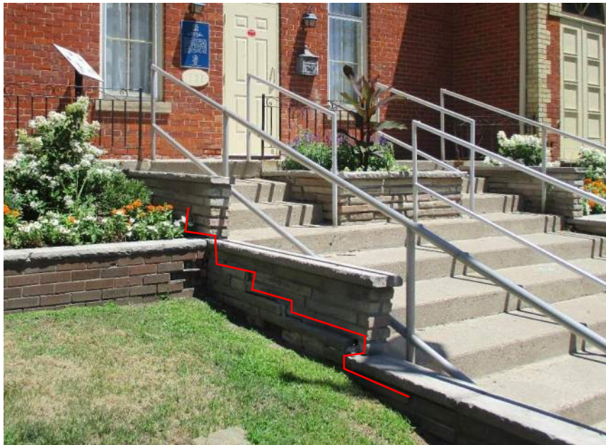
Photo # 16: View of displaced/cracking northern brick masonry low landscaping wall at the west elevation main entrance.
