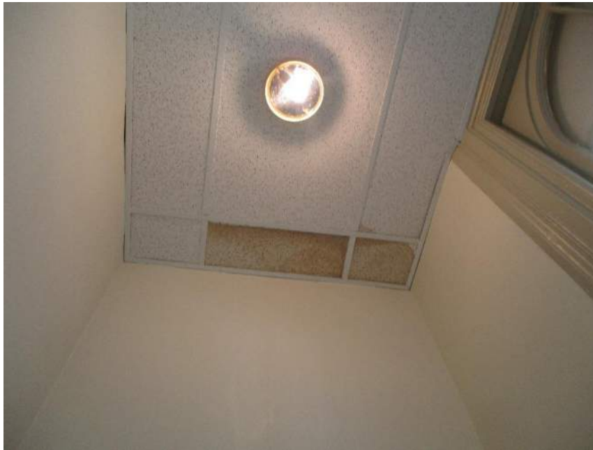
Photo # 23: View of stained ceiling tile in the women's washroom (north elevation, west addition).
