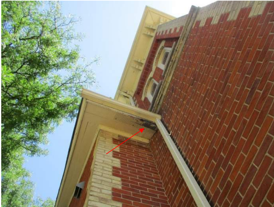
Photo #15: Typical view of localized area of soffit deterioration at the north elevation (west addition).
