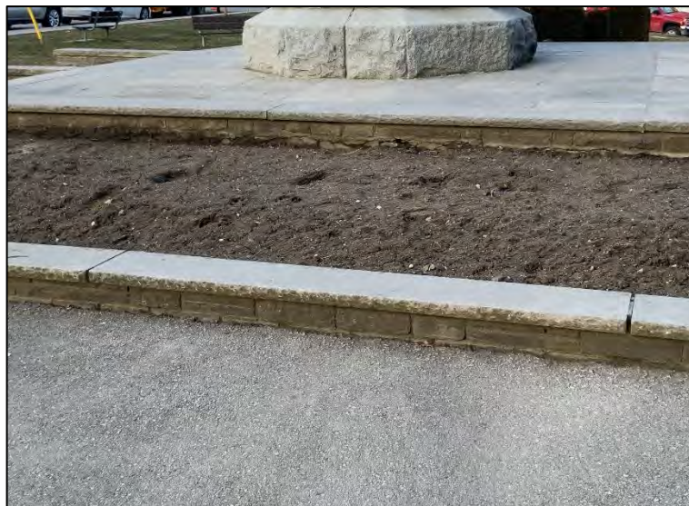
Photograph 3: Failed joints between capstones (Photo taken Jan. 2020)
