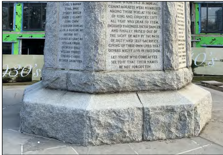
Photograph 1: Open joints in cenotaph base (Photo taken Jan. 2020)
