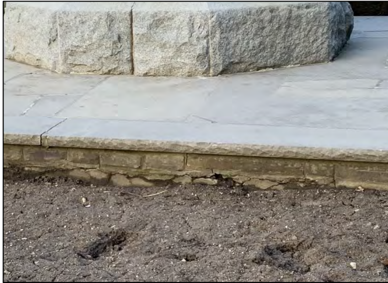
Photograph 2: Deteriorated horizontal joint at grade (Photo taken Jan. 2020)
