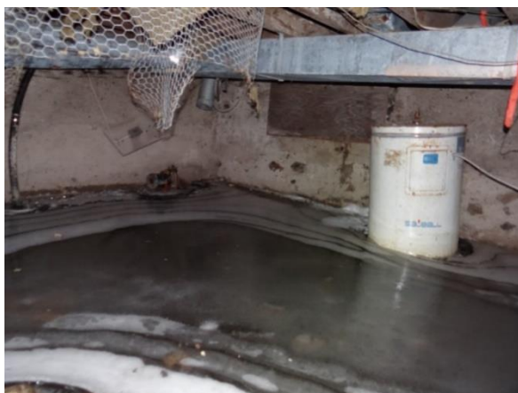
Plate 29: Detail of flooded basement.
