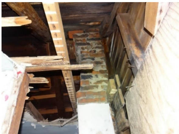
Plate 39: Detail of the chimney from the second floor to the exposed ceiling.
