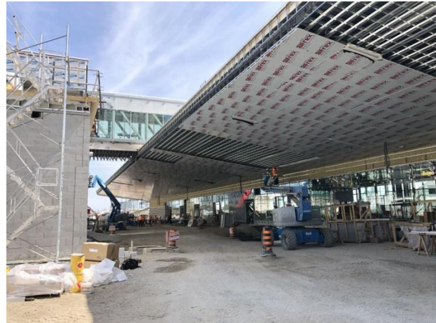
Terminal building (east view)
