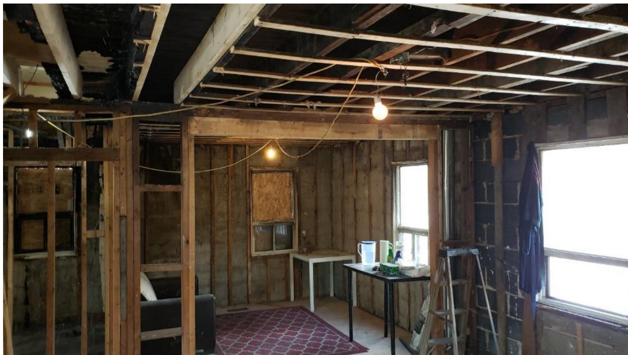
Figure 23 Interior fire damage, 40 Peter Street South. (Photo from client.)
