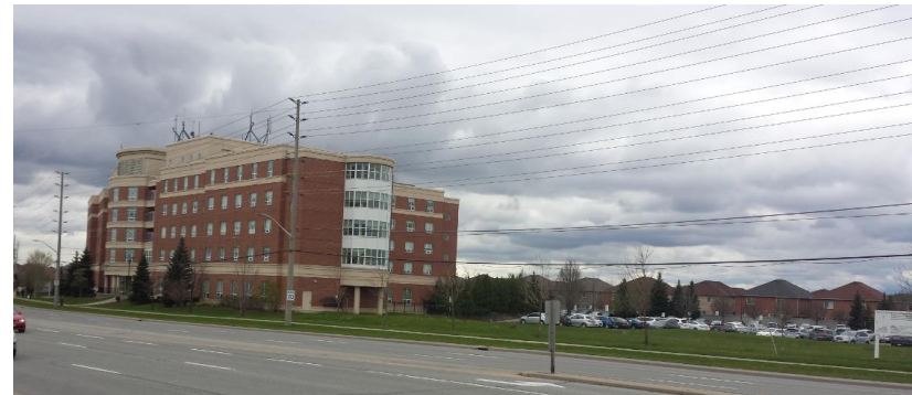
Image of existing conditions facing southwest (Mavis Road)
