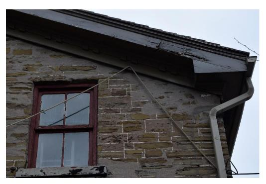
Image 6: Example of decay of underlaying substrate resulting from water exposure, due to a lack of preventative maintenance. All wooden surfaces exhibit similar signs of paint failure and decay.
