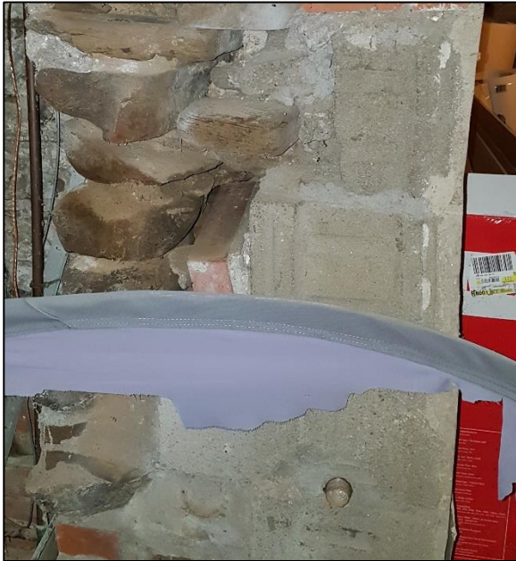
Figure 84: Photo of the stone foundation of the original building where it meets the concrete block foundation of the rear addition
