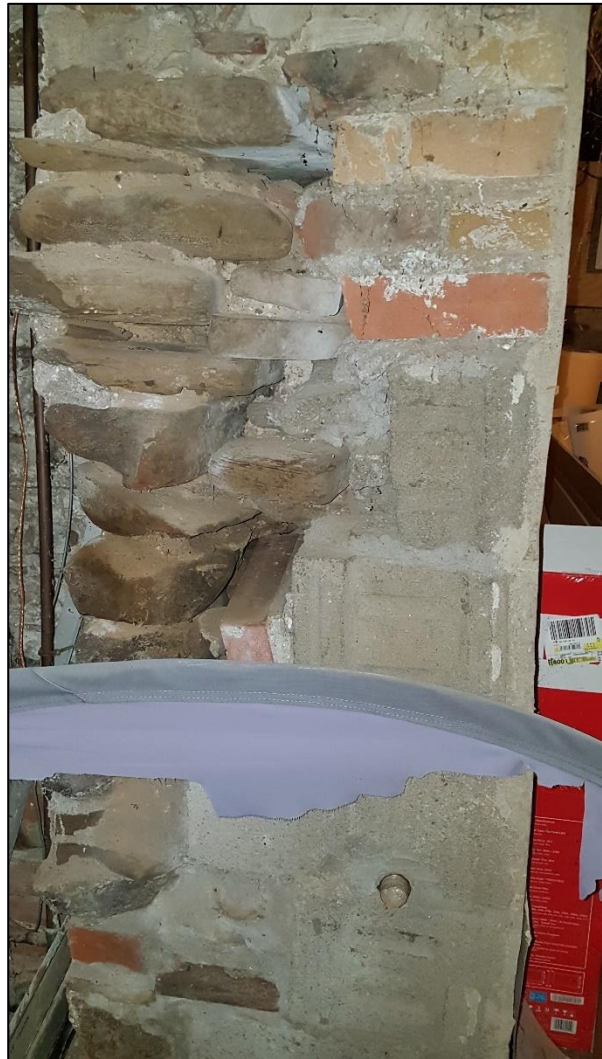
Figure 71: Portion of the foundation wall where the original stone foundation meets the concrete block foundation of the rear addition (note that portions have been repaired with brick)
