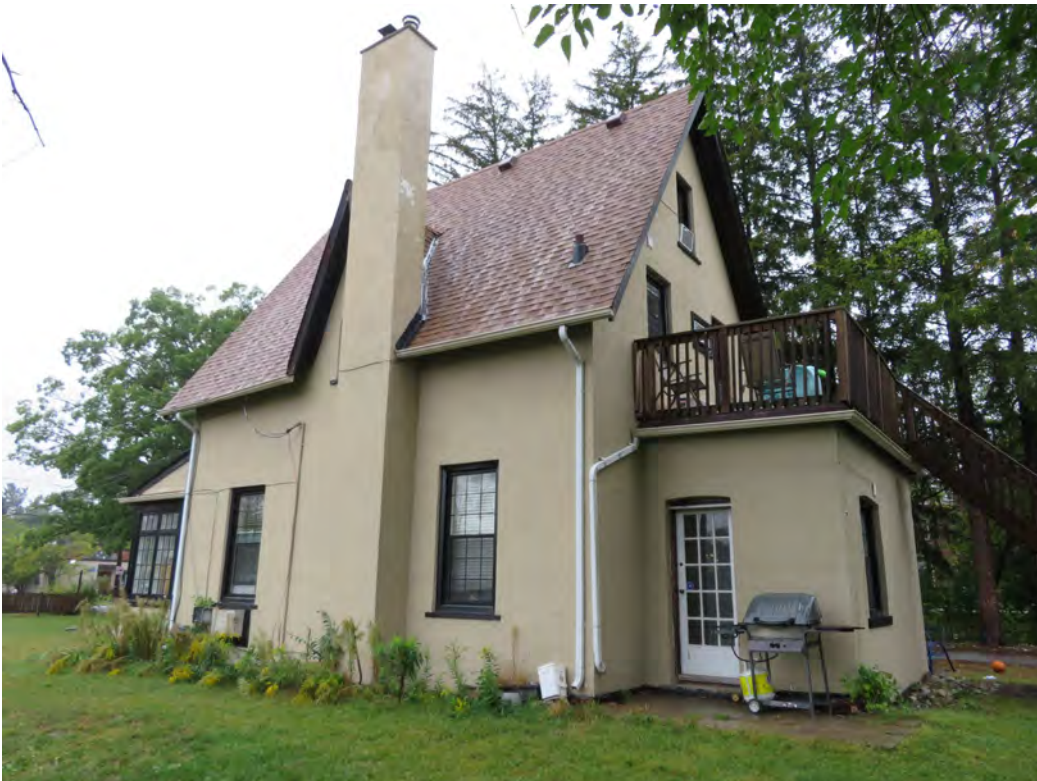
4.0 SOUTH ELEVATION – original front elevation - later chimney and 1-storey rear addition
