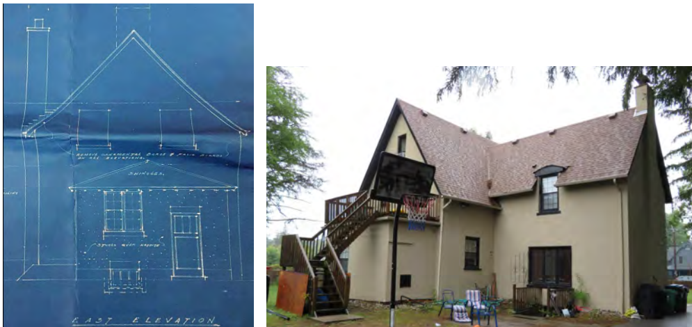
EAST ELEVATION – the 1936 rear addition corresponds to the 1936 blueprints but it now has a roof deck instead of a hipped roof – the large addition on the north side is a later alteration
