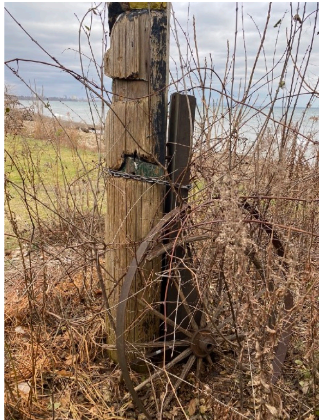
Photo 7: Steel beam and chain supporting base of pole.
