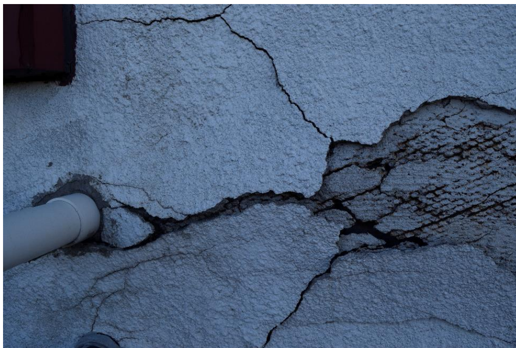
Image 6: Cracked and failing stucco on main façade.
