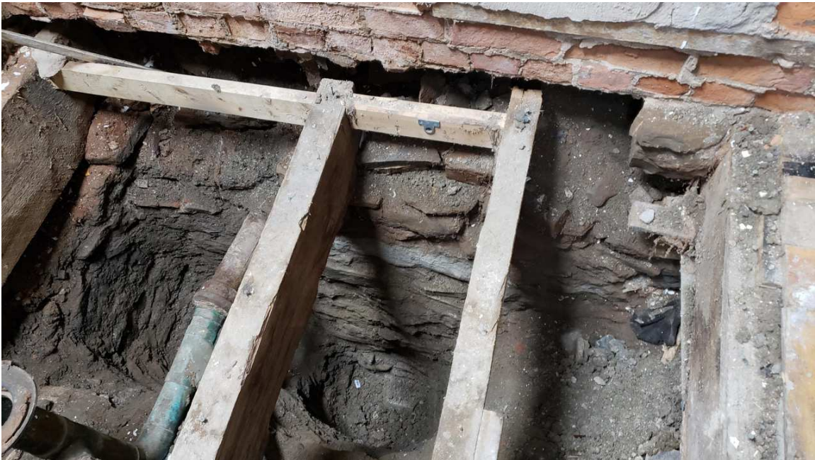
FOUNDATION – preliminary investigation of the footings
