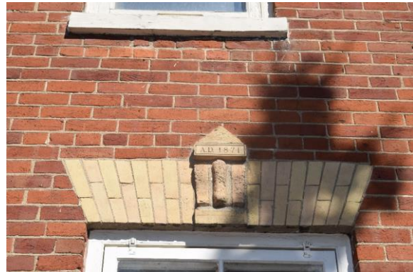
Plate 34: West elevation lower storey window with date keystone
