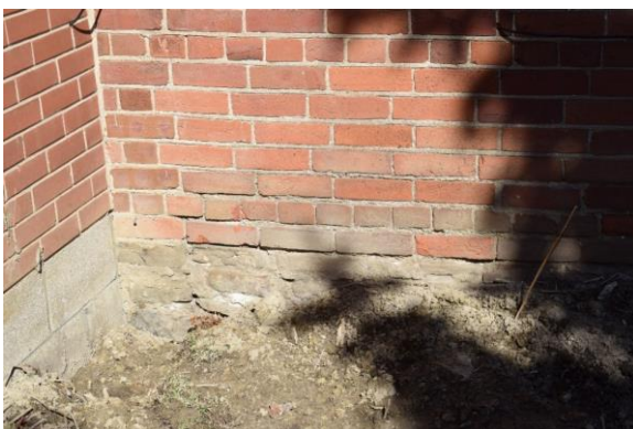
Plate 35: Stone foundation on west elevation
