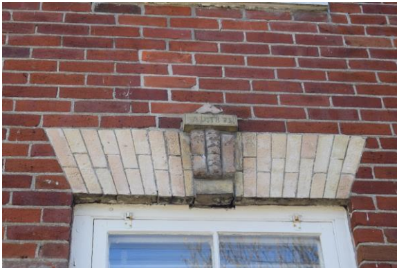
Plate 28: Close-up of date keystone above west window on east elevation
