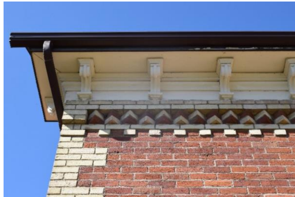
Plate 18: Close-up of eaves, moulded frieze, brackets, and dichromatic brickwork
