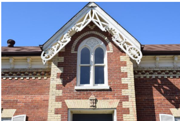
Plate 19: Bargeboard gable and Tuscan Gothic window looking north
