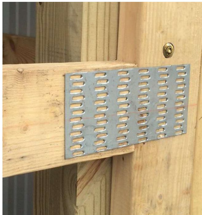
GANG NAIL PLATE USED TO CONNECT TWO PIECES OF WOOD (STOCK PHOTO)
