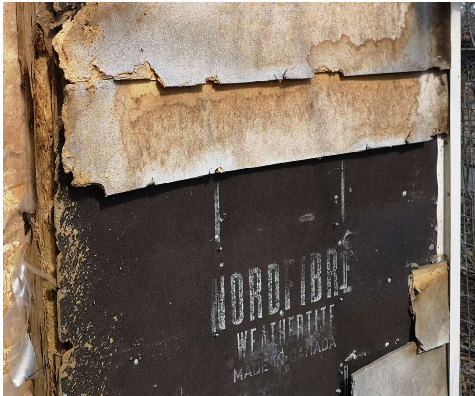
DETAIL OF SHEATHING MATERIAL. NOTE REMNANTS OF ORIGINAL FIBER SIDING MATERIAL
