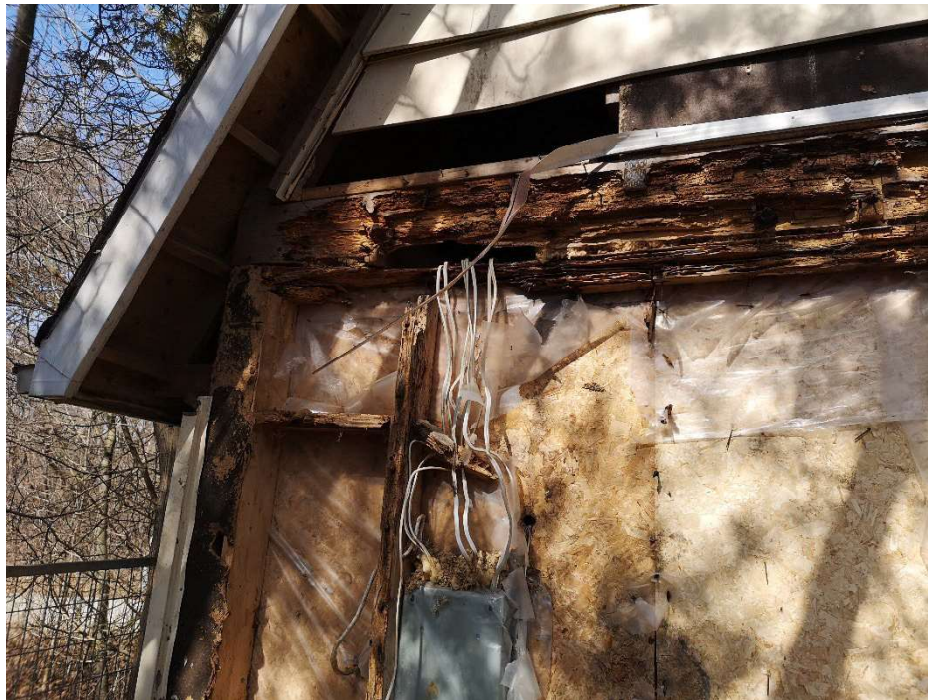
SIGNIFICANT ROT OF FRAMING MEMBERS ON REAR ELEVATION
