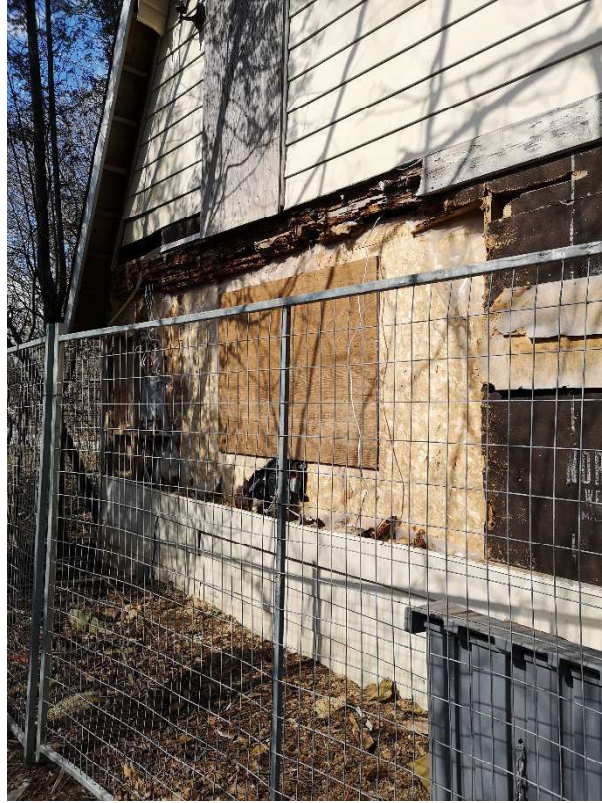
DETERIORATION AND REMOVAL OF MATERIALS ON REAR ELEVATION
