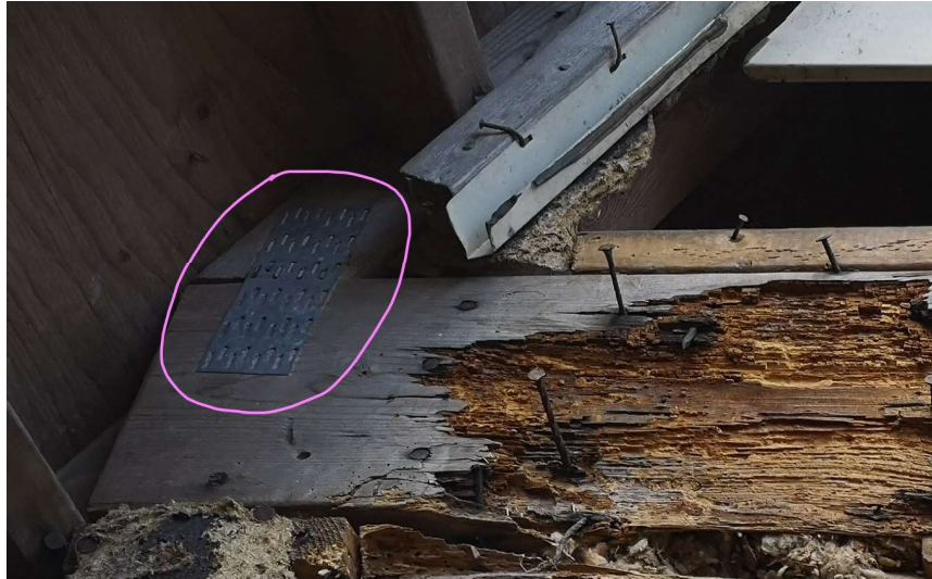
GANG NAIL PLATE VISIBLE ON REAR ELEVATION OF GARAGE
