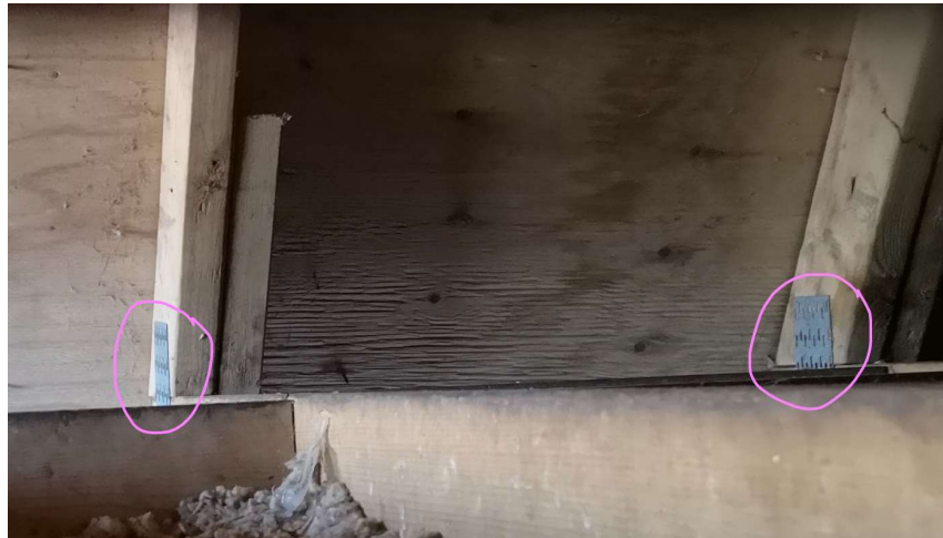
GANG NAIL PLATES VISIBLE FROM INTERIOR ON NORTH WALL
