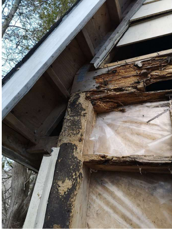
DETAIL SHOWING ROTTED MEMBERS, NEWER ROOF FRAMING, ALUMINUM SIDING AND FASCIA
