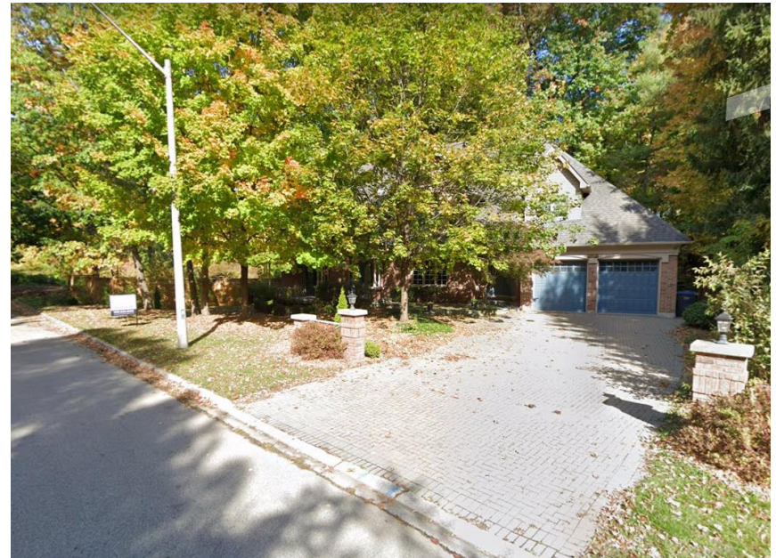
Image of existing conditions facing northeast
