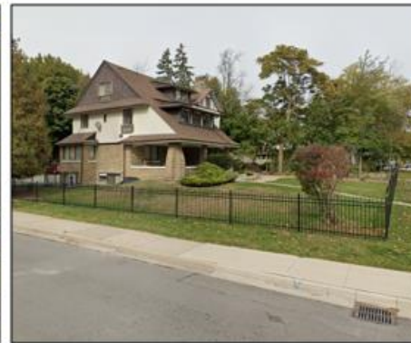
Looking northeast at heritage designated building to be retained (contains 6 apartment units)
