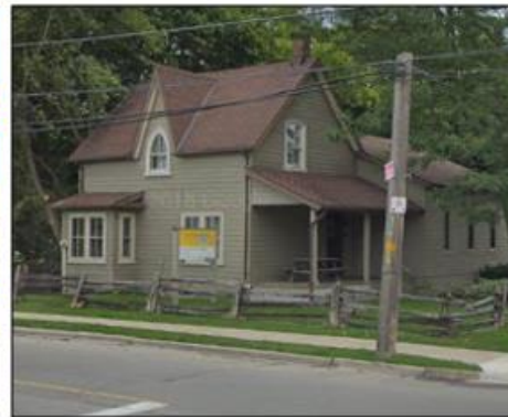
Looking southeast (building to be redeveloped)
