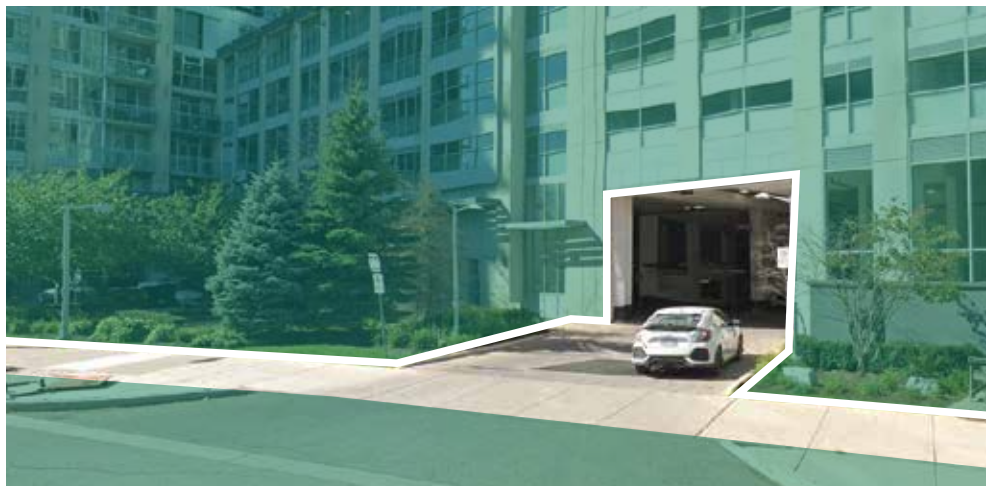
Figure 22: Provision for vehicular access to off-street parking, access for deliveries, garbage pick-up, servicing and loading. Downtown Mississauga, Webb Dr & Duke of York Blvd
