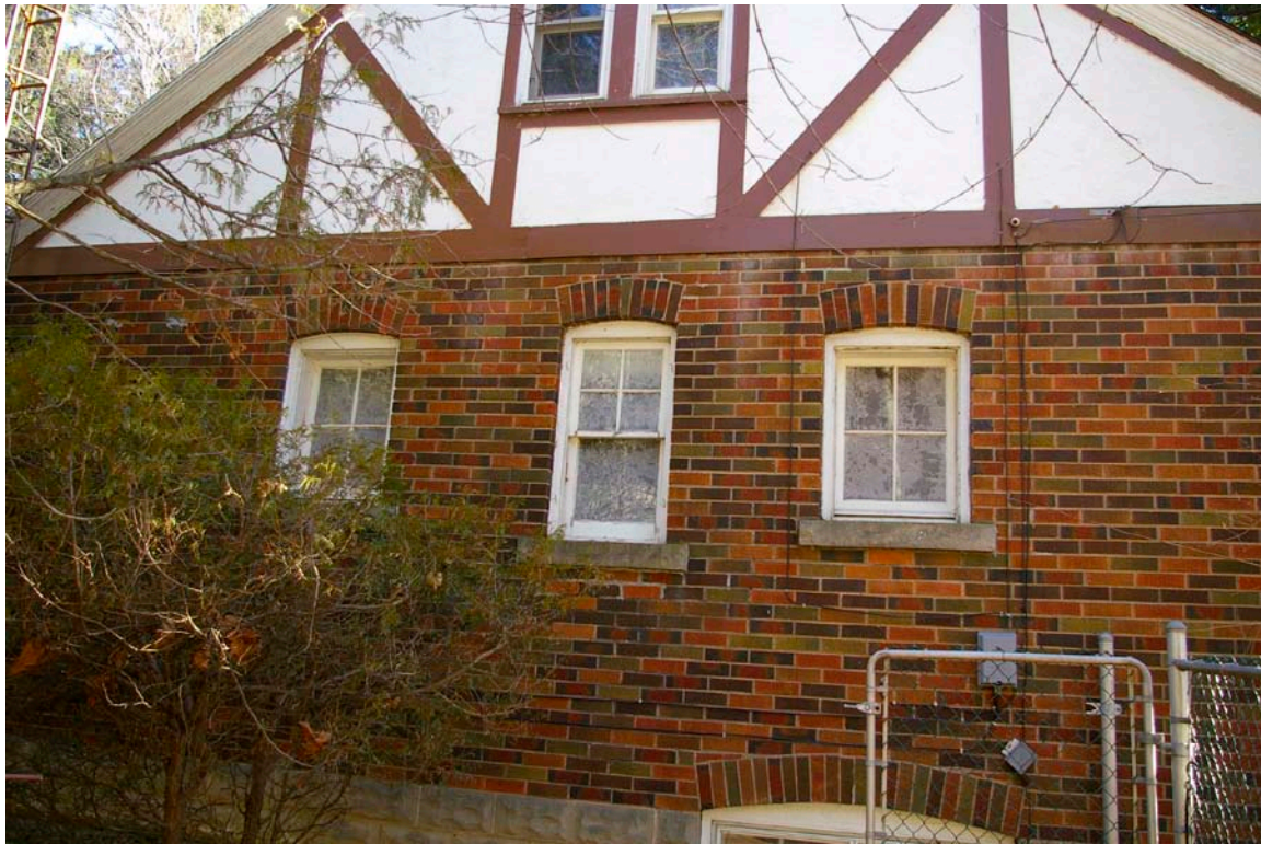
Photo 31 West façade showing the rug brick masonry veneer and segmental arches over the windows. Foundation walls above grade constructed of rock-faced concrete block. The small windows are in the two bedrooms on the west side; centre window is for a bathroom.
