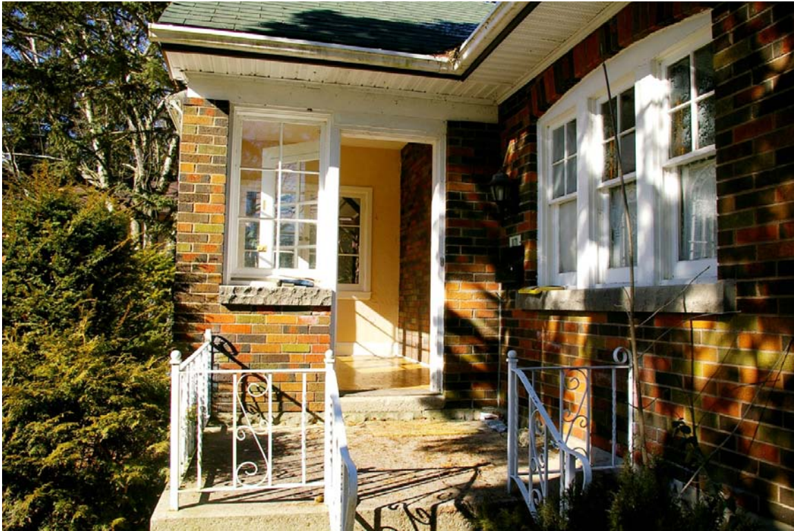
Photo 29 View looking across the concrete landing into the entrance porch. Window lintels constructed of poured concrete with a rock face.
