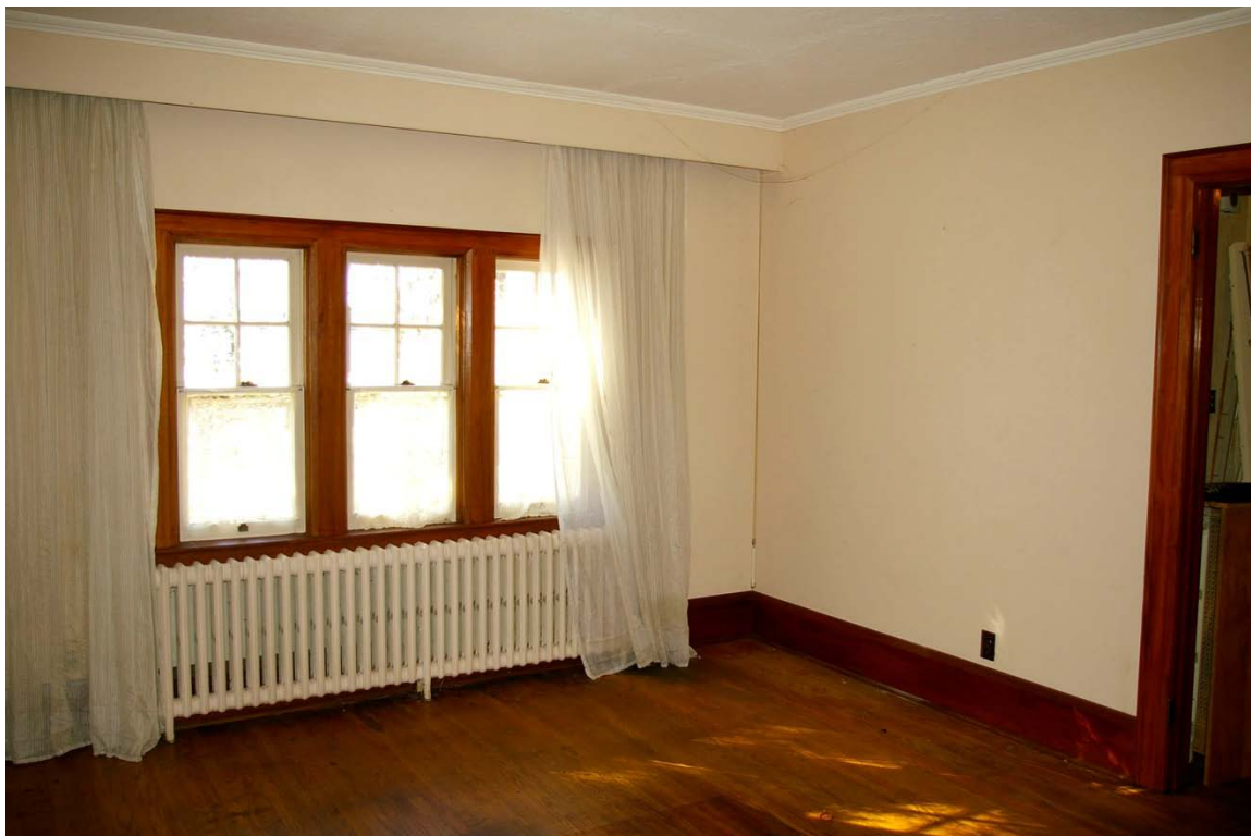
Photo 46 Living room with doorway from the hallway to the right. Shows one of numerous cast-iron radiators for the hot water heating system and the original hardwood flooring and varnished wood baseboards and trim in the living and dining rooms.
