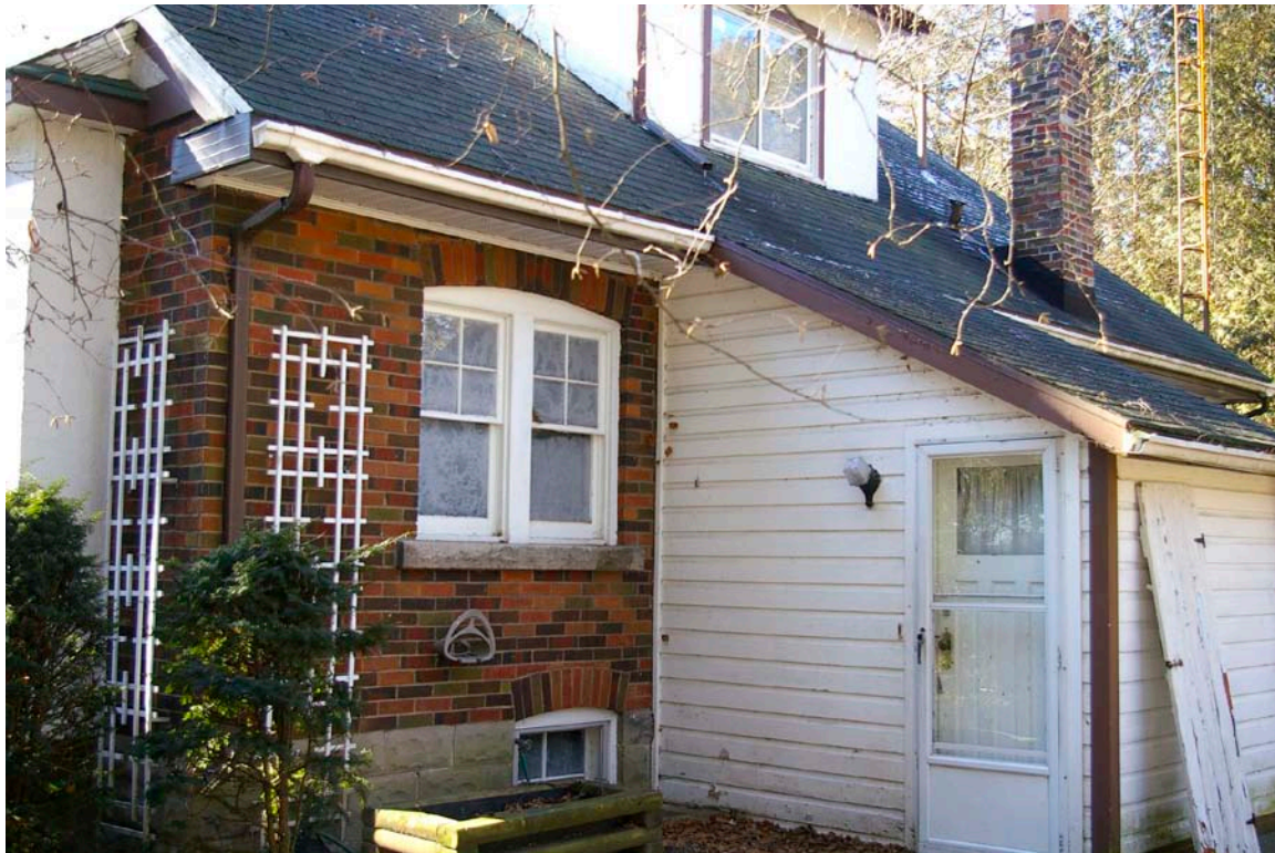
Photo 35 Rear façade showing the entrance to a rear addition clad in shiplap horizontal wood siding with an aluminum storm door (possibly a replacement for solid door leaning against the rear wall) and the original wood panelled and glazed door.
