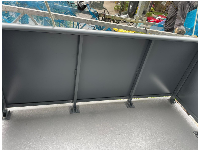
Full Height Aluminum Panel Guard - Colour to be Washington White to match existing balcony guards
