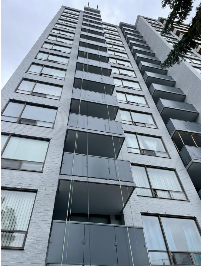
Full Height Aluminum Panel Guard - Colour to be Washington White to match existing balcony guards
