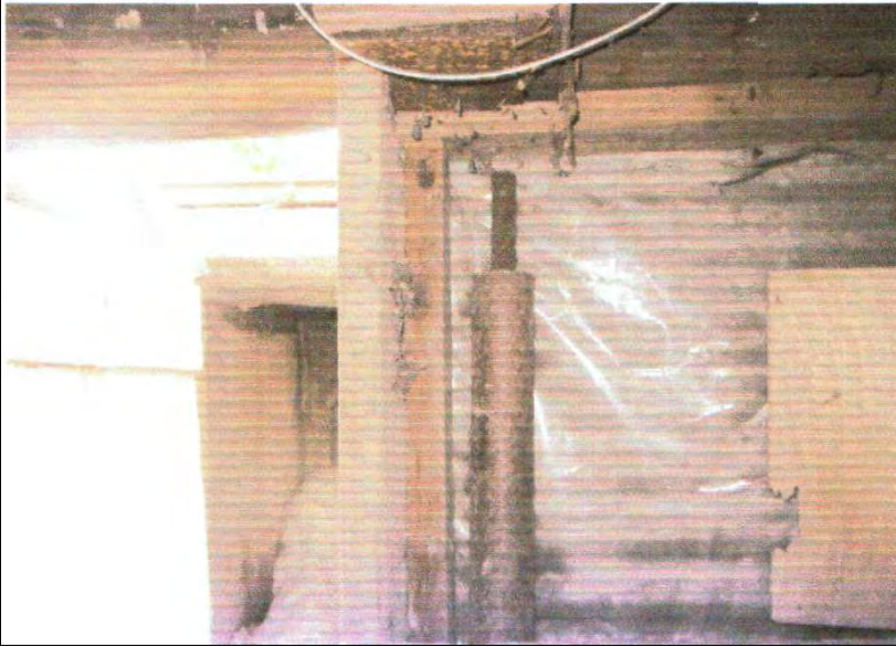
Figure 17 damaged support beam & post, temporary post missing top plate
