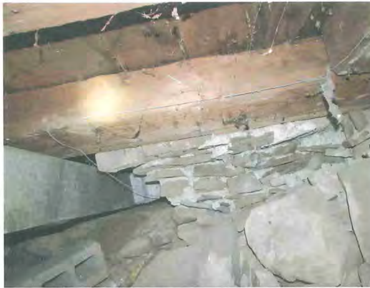
1880s foundation beyond 1840s timber sill plate
