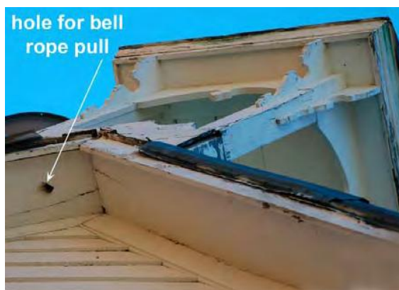
Figure 25 bell tower with bell rope pull hole
