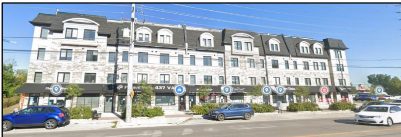
551 Lakeshore Road East
