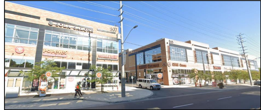
507-515 Lakeshore Road East
