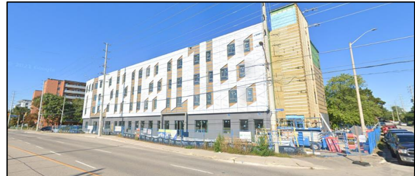
425 Lakeshore Road East
