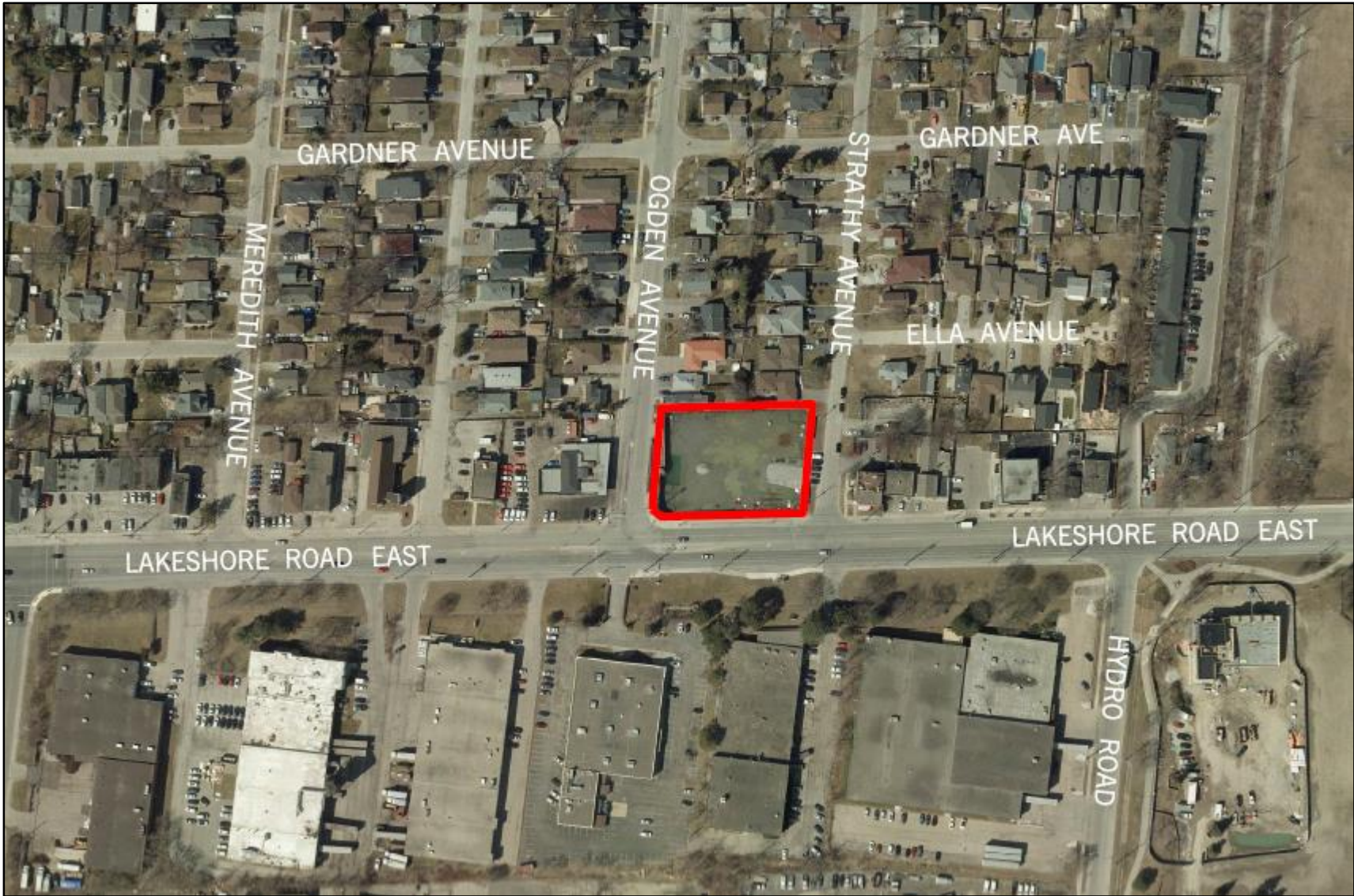
Aerial Photo of 1041 Lakeshore Road East
