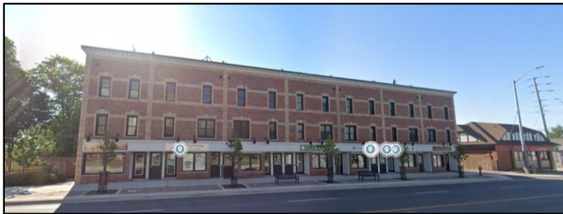
760 Lakeshore Road East
