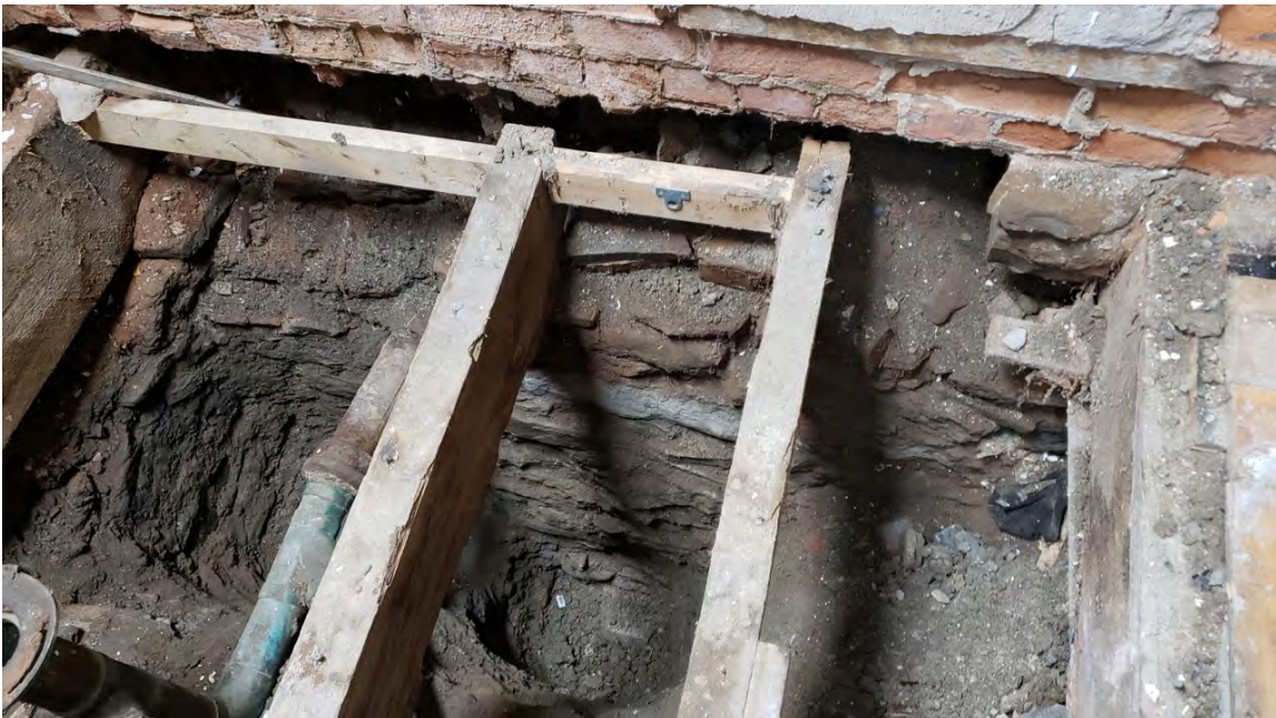
FOUNDATION – preliminary investigation of the footings
