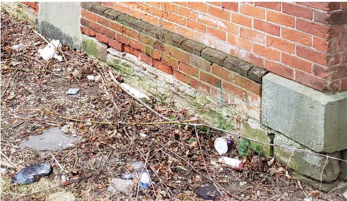
EXTERIOR – rubble stone foundation
