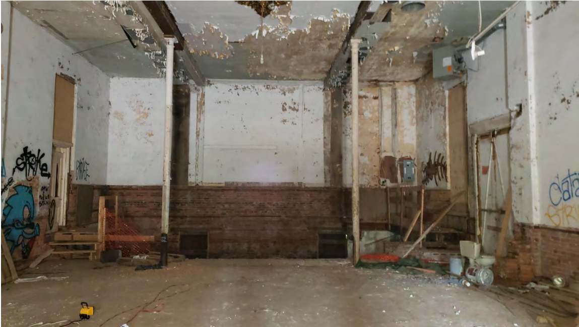
INTERIOR – 1 st FLOOR – 2 cast iron columns are original
