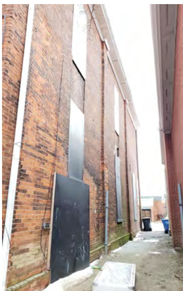
EXTERNAL FIRE EXIT STAIR – a free-standing exit stair will be built on the north side in the alleyway - a window on the 2 nd floor will be modified for a new door
