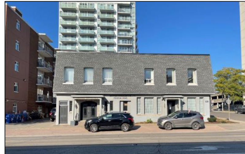
Image of existing condition facing northwest from south of Lakeshore Road East
