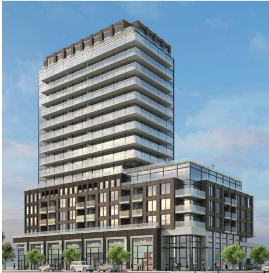
Applicant's rendering of the proposed apartment building with ground floor commercial uses (facing northwest at Lakeshore Road East and Elmwood Avenue North)
