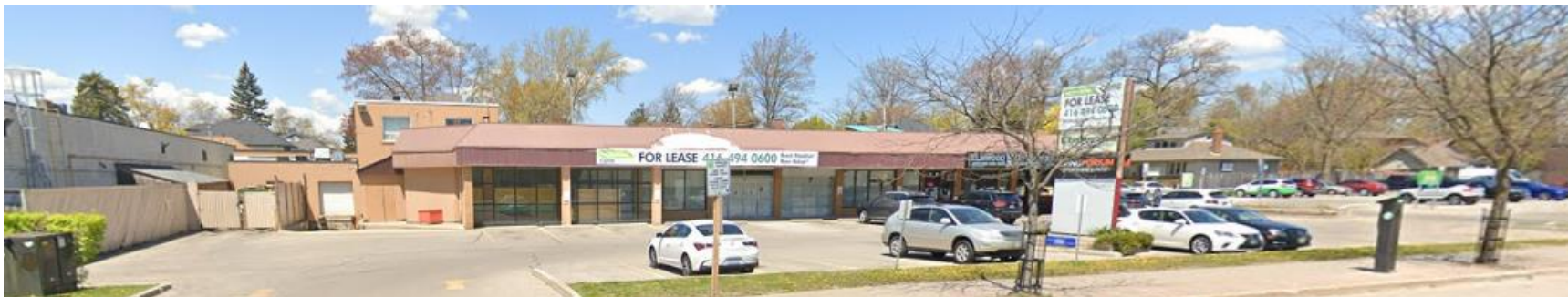
Existing Conditions – facing north from Lakeshore Road East
