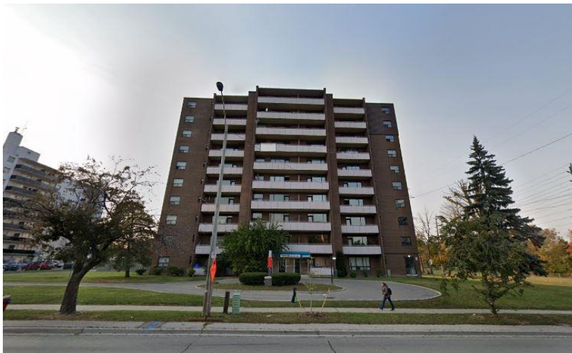
Image of existing conditions facing north
