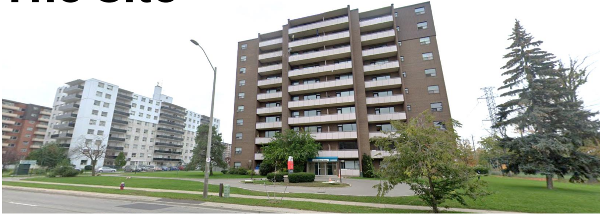
Views looking north of Bloor Street (front of building)
