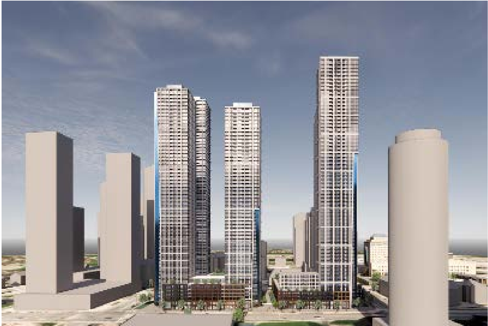
View facing north (Burnhamthorpe Road West frontage)
