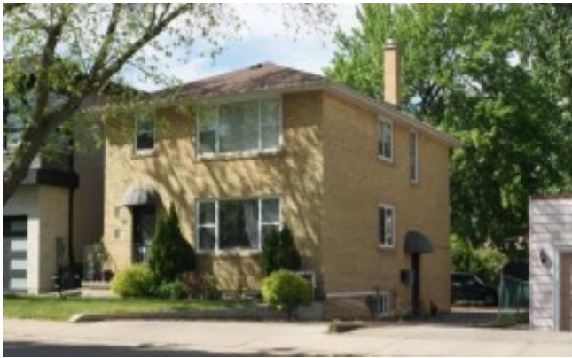
Existing triplex conversion
