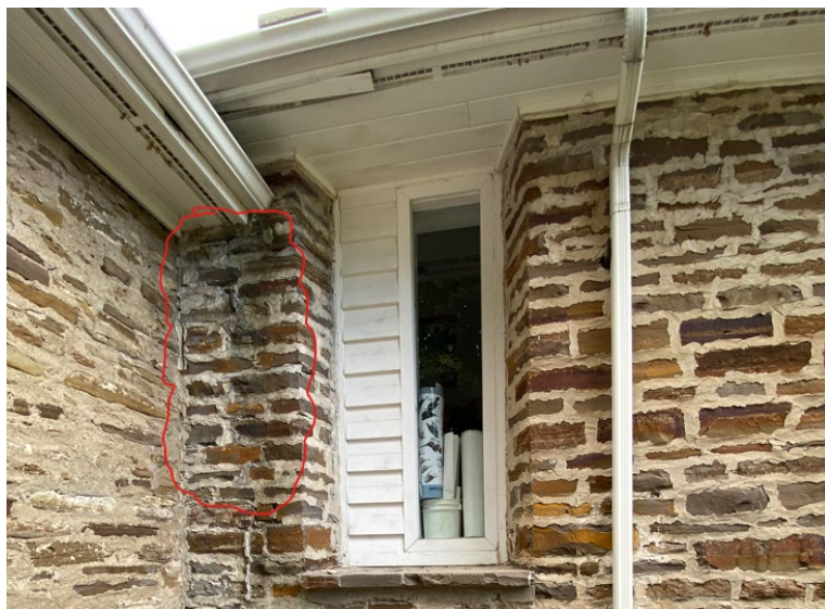
Example of Wall Deterioration Apparently Caused by Poor Eavestrough Detailing or Condition
