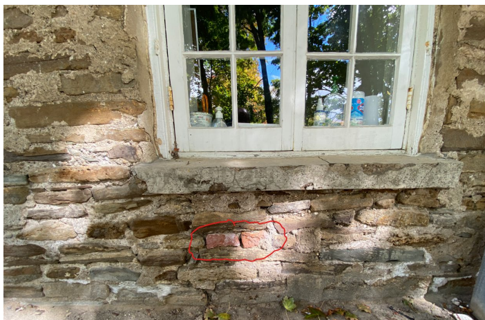
Example of Brick Fragment in Existing Stone Wall
