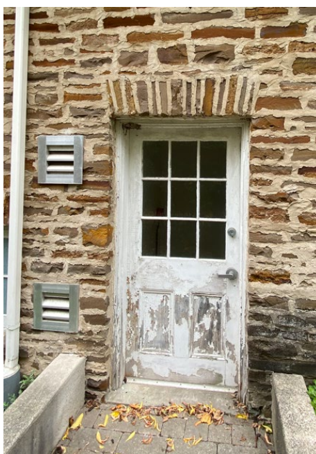
Example of Deteriorated Paint Finish on Exterior Door and Frame
