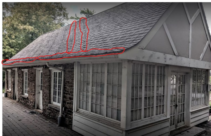
Note Shingle Deterioration along Lower Edge of Roof, Diagonal Banding on Roof from Curling of Shingles
