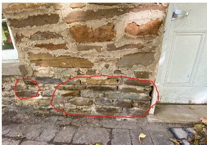
Note Deteriorated and Missing Mortar
