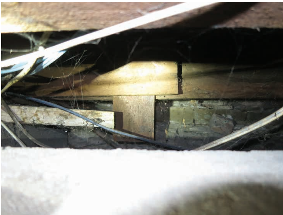
Exposed rubble foundation wall (ERA, 2022).
