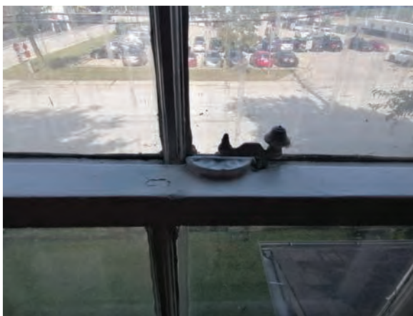
Detail of north elevation second storey window showing sash lock (ERA, 2021).
