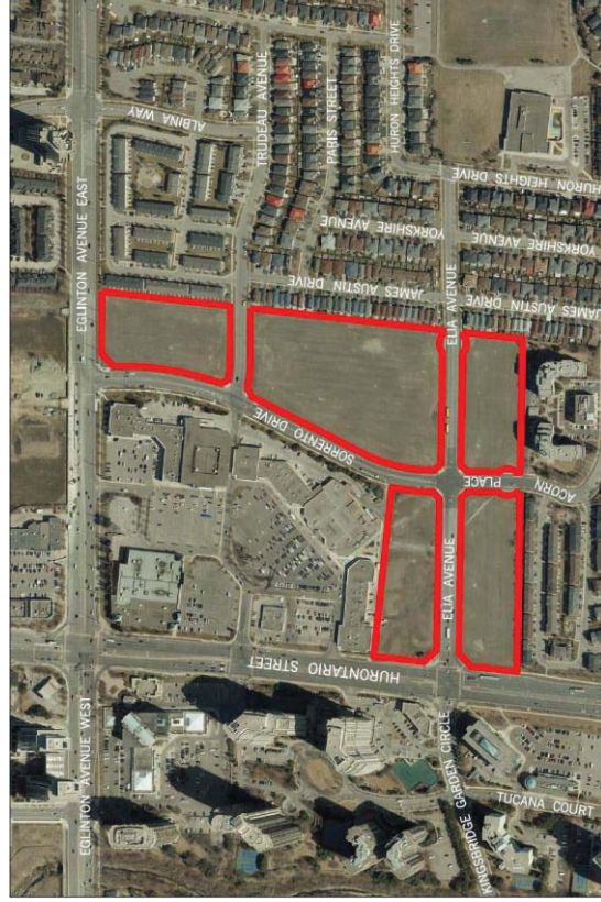
Aerial Photo of 4615 Hurontario Street, 25, 35, 55, 105 and 110 Elia Avenue and 136 Eglinton Avenue East
