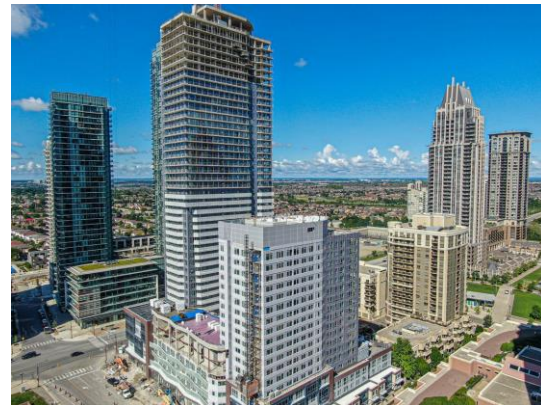
#6 – Support Region of Peel affordable housing projects (example: 360 City Centre Drive)
