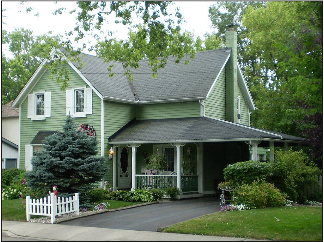
3.1.3d: Steven Lester Peer residence (42 John Street South), built 1897
