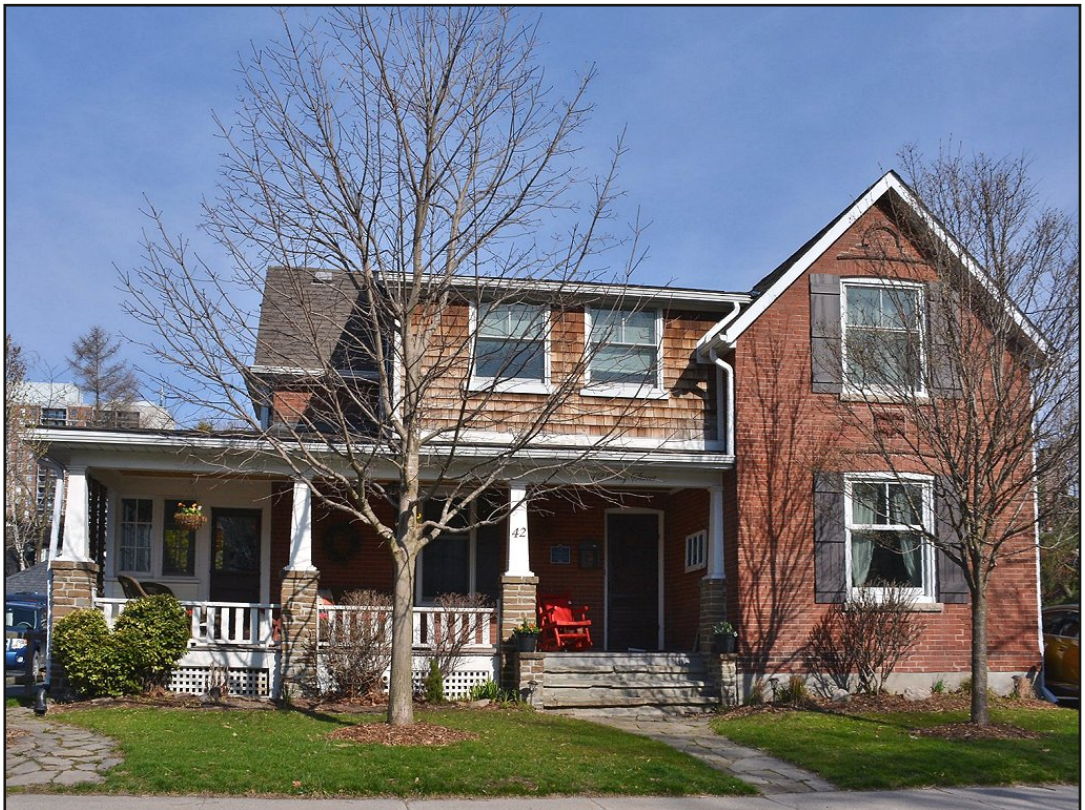
2.4.3d: property west of the subject property (42 Bay Street)
