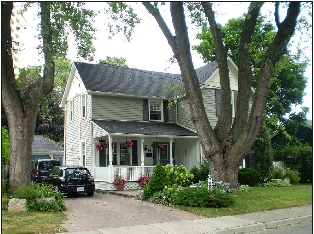
3.1.3c: Cpt. Albert E. Block residence (39 John Street South), built 1912
