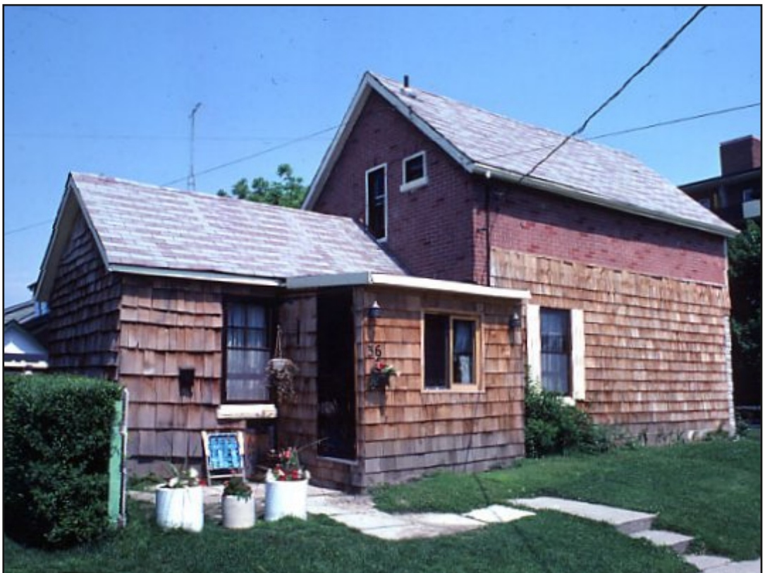
2.3.6e: south and west elevations, ~1980
