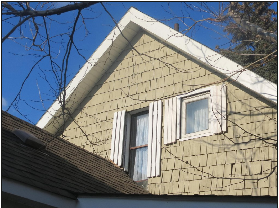
2.3.2h: first generation windows and shutters
