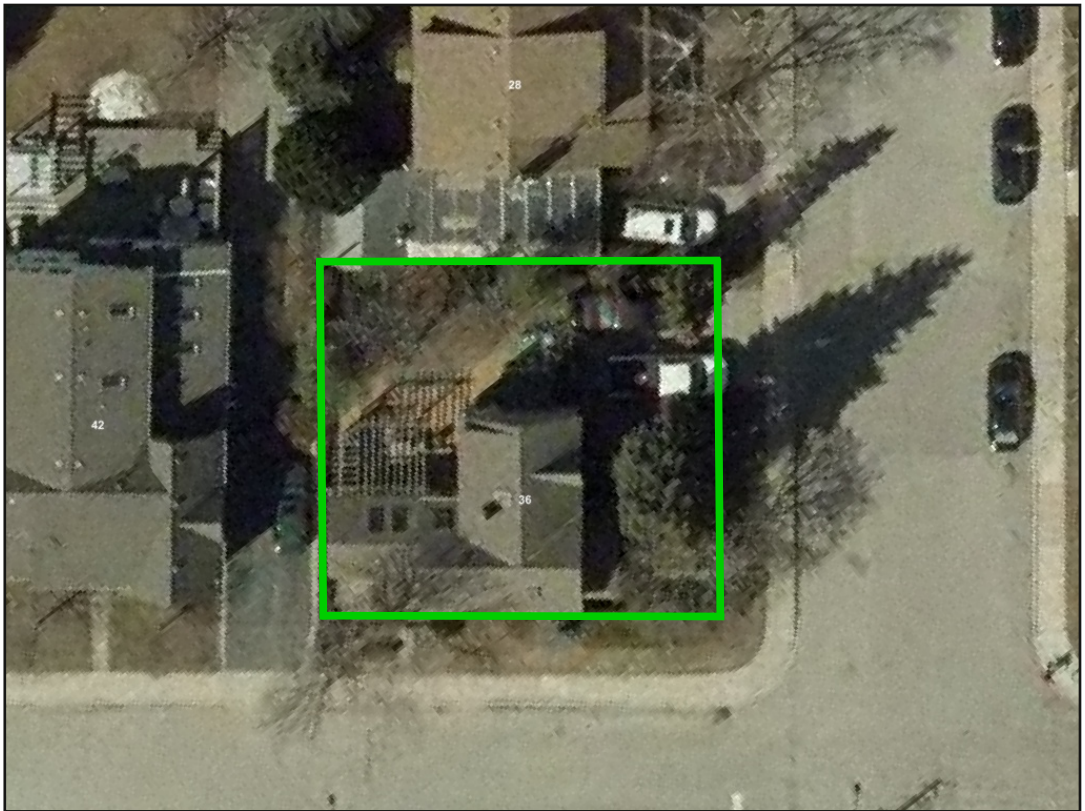
2.2.3a: 2021 aerial image (City of Mississauga)
