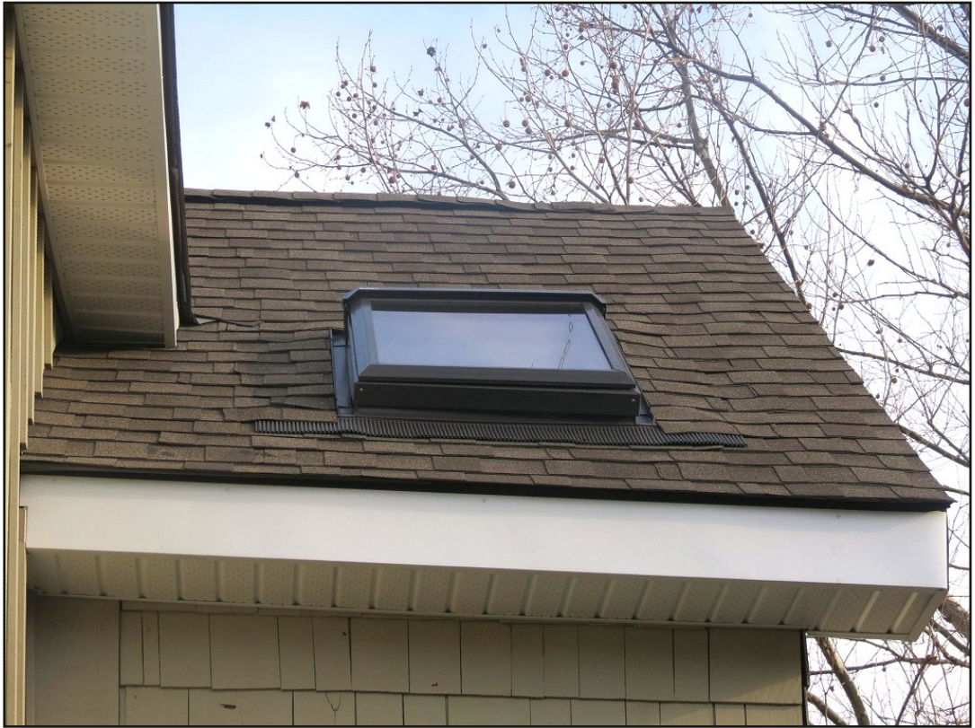
2.3.2g: skylight window
