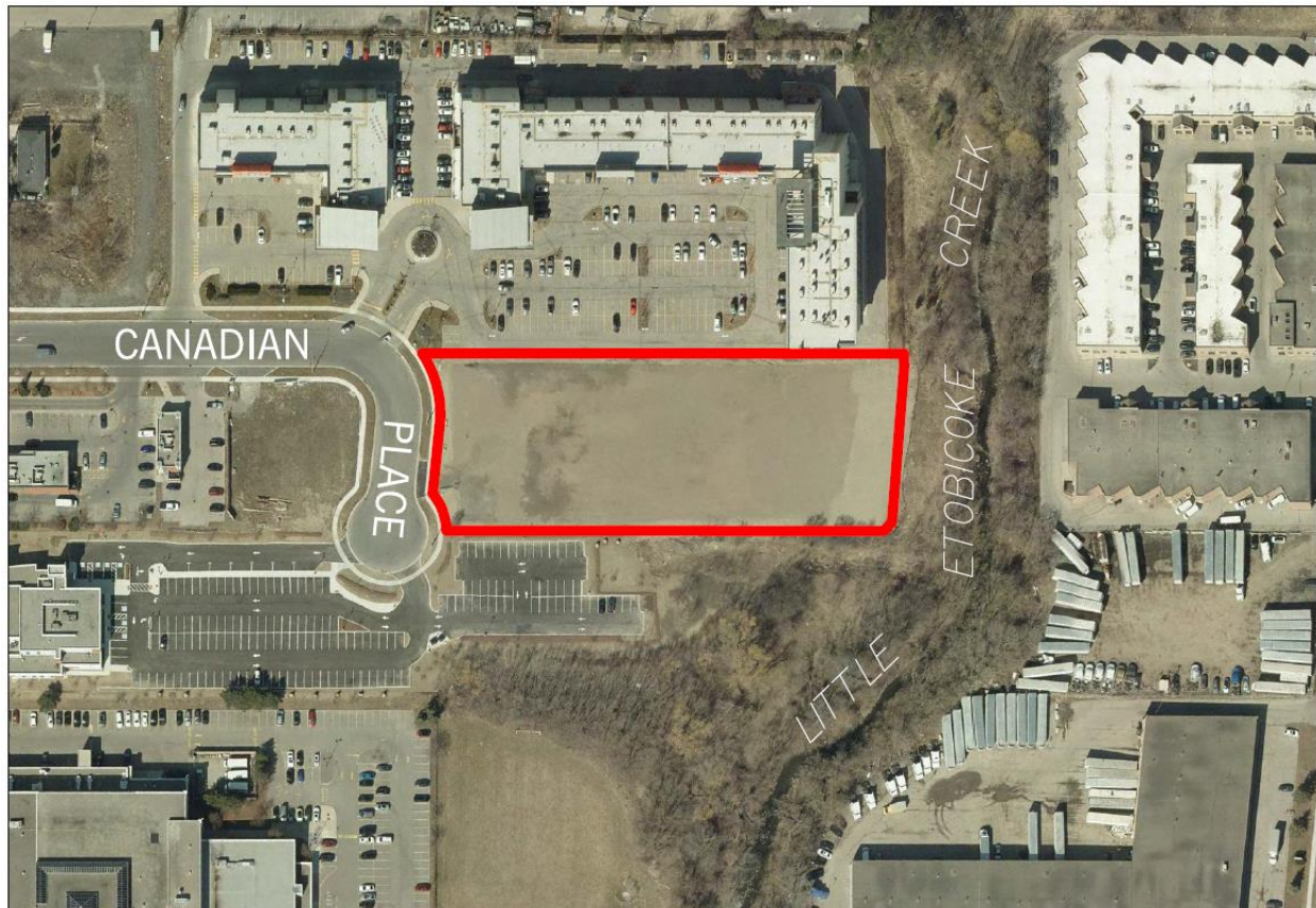
Aerial Image of 1075 Canadian Place
