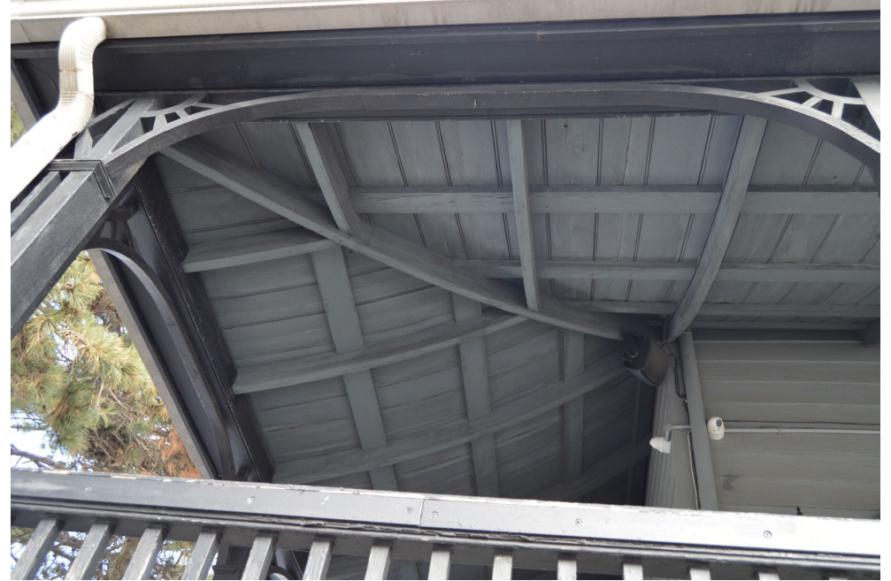
Fig. 27 A close-up view of the underside of the verandah roof
