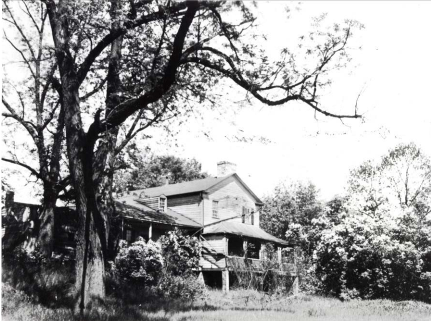
Fig. 8 Arthur Malcolm Mushlian, "Cherry Hill House, Dixie," c. 1930, Mississauga Library System, I.D. MC0002. A side view of the house shows the bent board-and-batten roof surmounting the verandah and asphalt shingle covering the roofs over both the front part and back wing.
