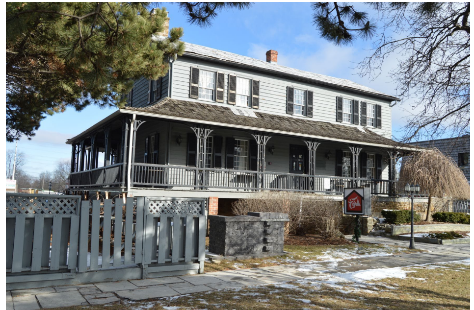
Fig. 19 Corner view, showing a portion of the house's north elevation and the front facade
