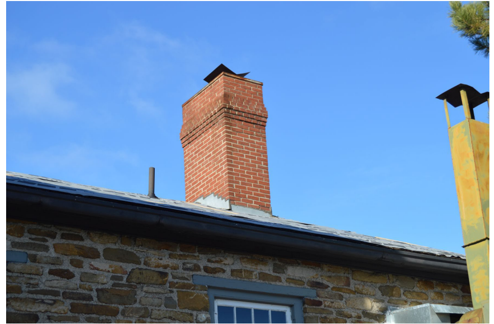
Fig. 31 Rebuilt red brick chimney on the back wing
