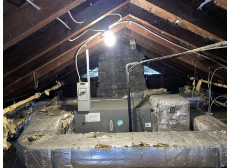
Fig. 37 View of the same attic, looking north to the stone chimney
