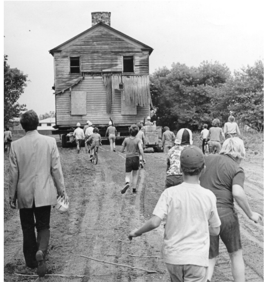
Fig. 15 The house in transit, 1973. Photo courtesy of Heritage Mississauga.
