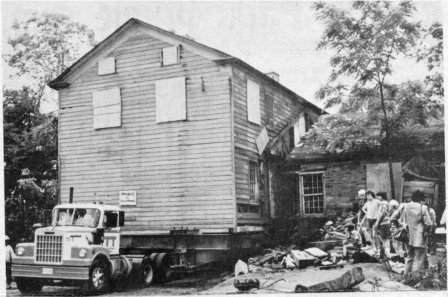
Fig. 14 Preparing Cherry Hill House for the move, 1973. Photo courtesy of Heritage Mississauga.
