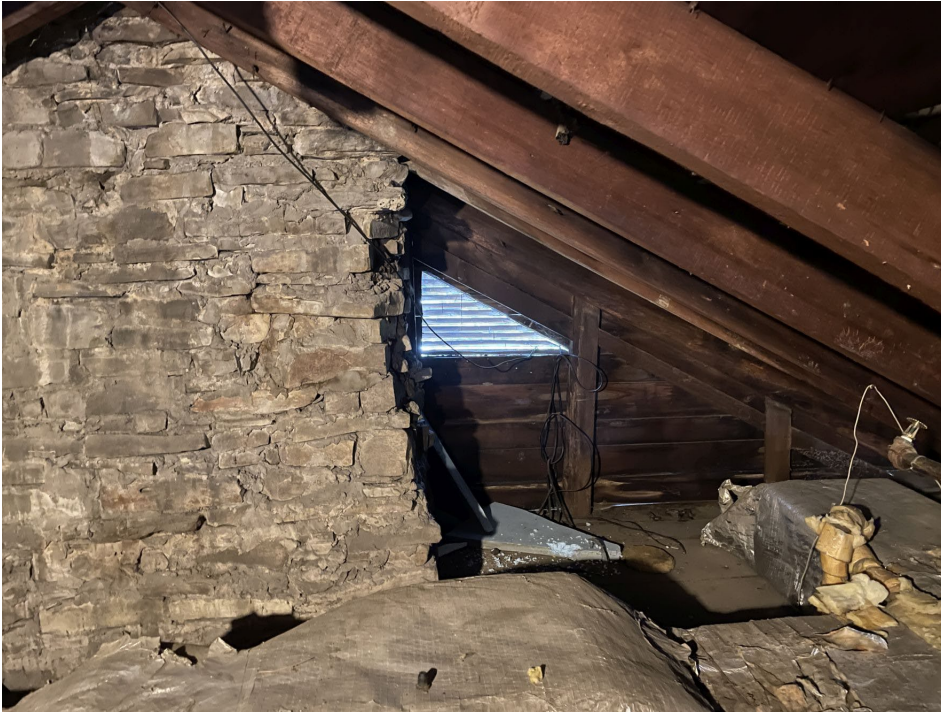
Fig. 38 North end of the same attic
