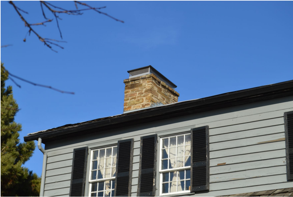
Fig. 30 Rebuilt stone chimney at the house's north gable end
