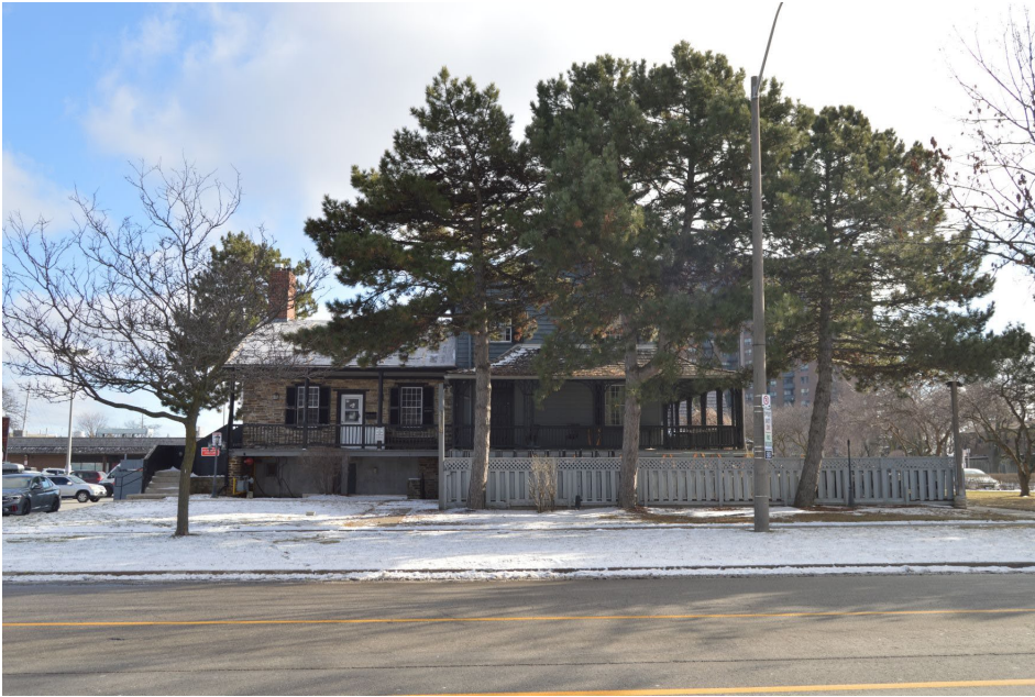
Fig. 20 North elevation facing Silver Creek Boulevard, hidden by Austrian pines and a contemporary wood patio screen enclosure
