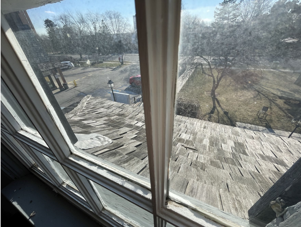
Fig. 32 View from inside the building, looking west over the verandah roof with its weathered silvery-grey wood shingle cladding
