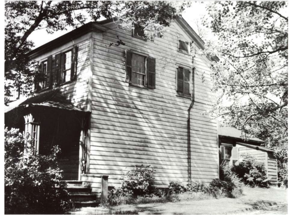
Fig. 7 Arthur Malcolm Mushlian, "Cherry Hill House, Dixie," c. 1930, Mississauga Library System, I.D. MC0005. The corner view of the front elevation and one side elevation shows the verandah's bent board-and-batten roof, then perhaps eight decades old.
