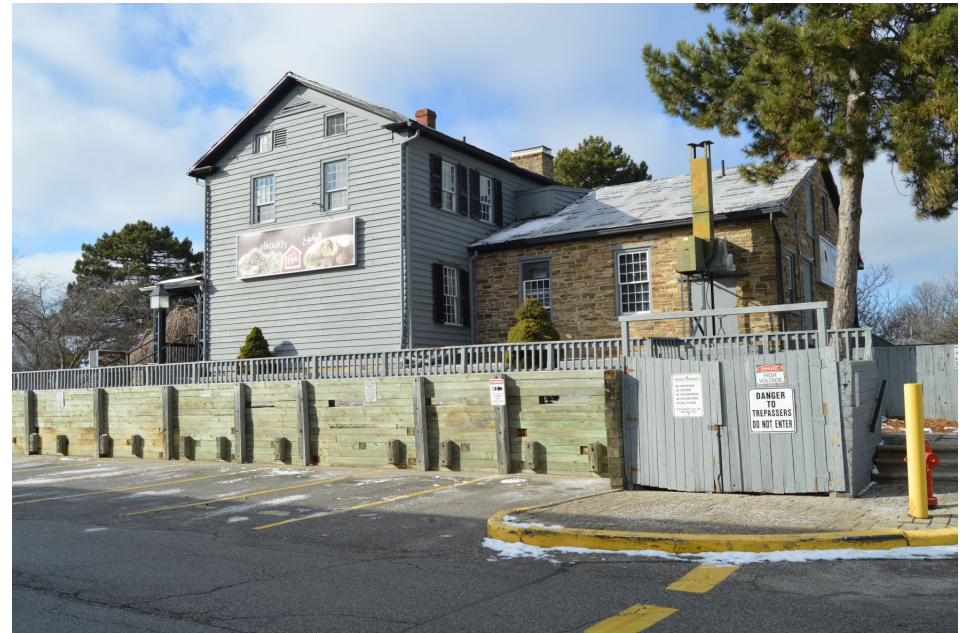
Fig. 23 Corner view, showing the south and rear elevations. The tarpaulin fitted over the back wing's gable roof is clearly shown. Note the unattractive wood screen enclosure for the mechanical equipment, the prominent metal vent on the back wing and another restaurant sign tacked onto the wall.
