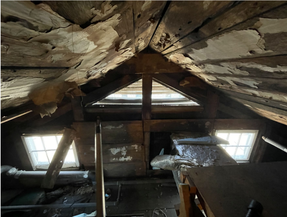
Fig. 36 South end of the same attic
