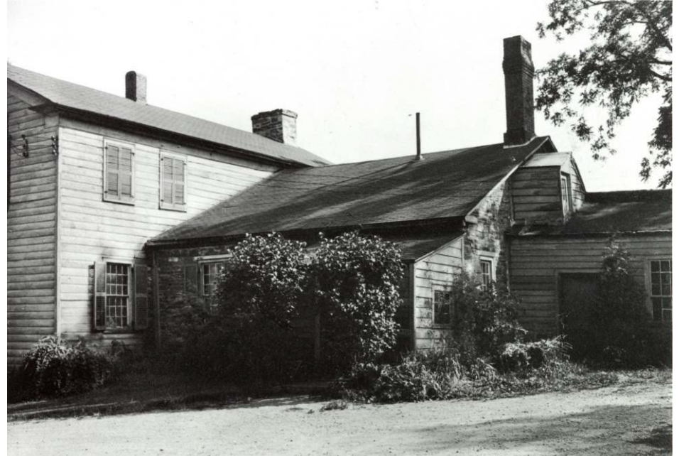
Fig. 9 Arthur Malcolm Mushlian, "Cherry Hill House, Dixie," c. 1930, Mississauga Library System, I.D. MC0003. The rear view shows asphalt shingle on the house's front part and back wings.
