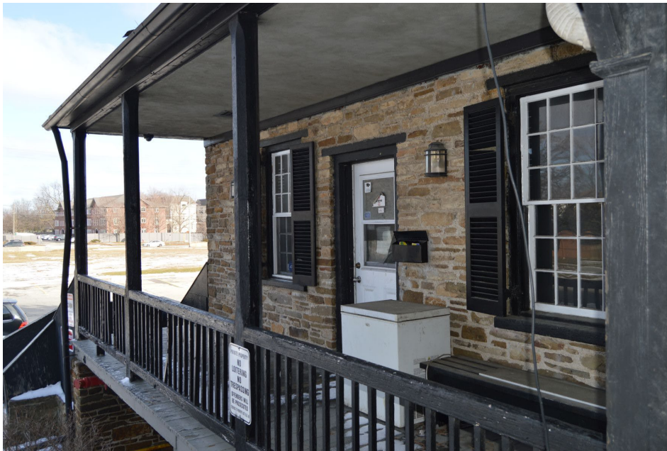
Fig. 28 View of the back wing's verandah in apparently good condition
