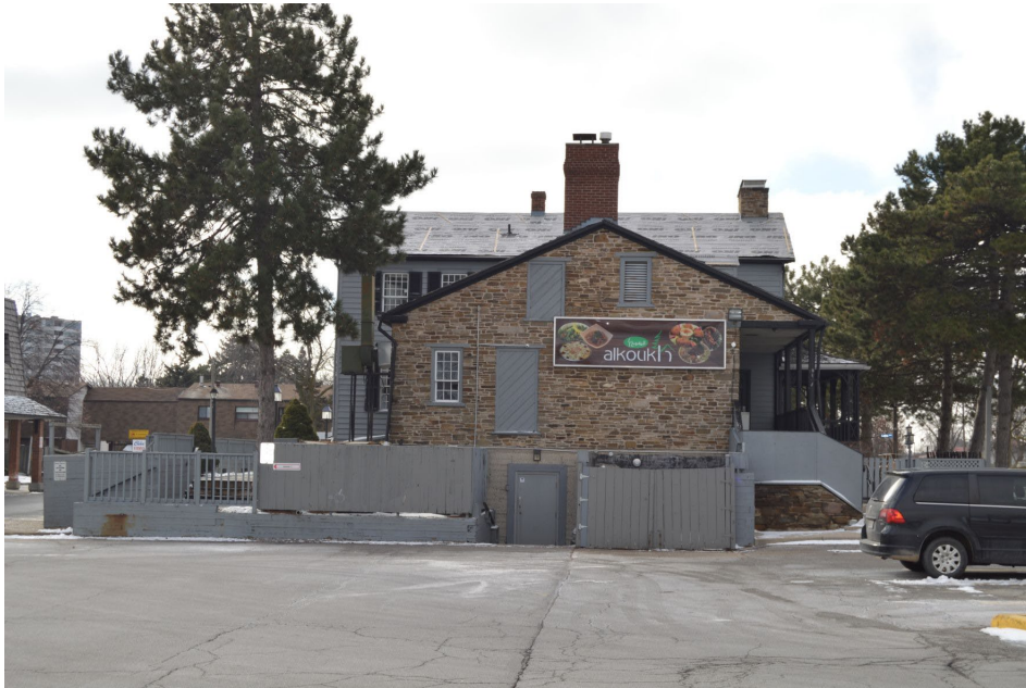
Fig. 22 East elevation facing the Silver Creek Plaza parking lot. Detracting from the elevation's visual appeal are the wood screen enclosures around the garbage collection area and mechanical equipment area, the solid balustrade along the stairs to the back wing's verandah and the large wall sign for the defunct restaurant.
