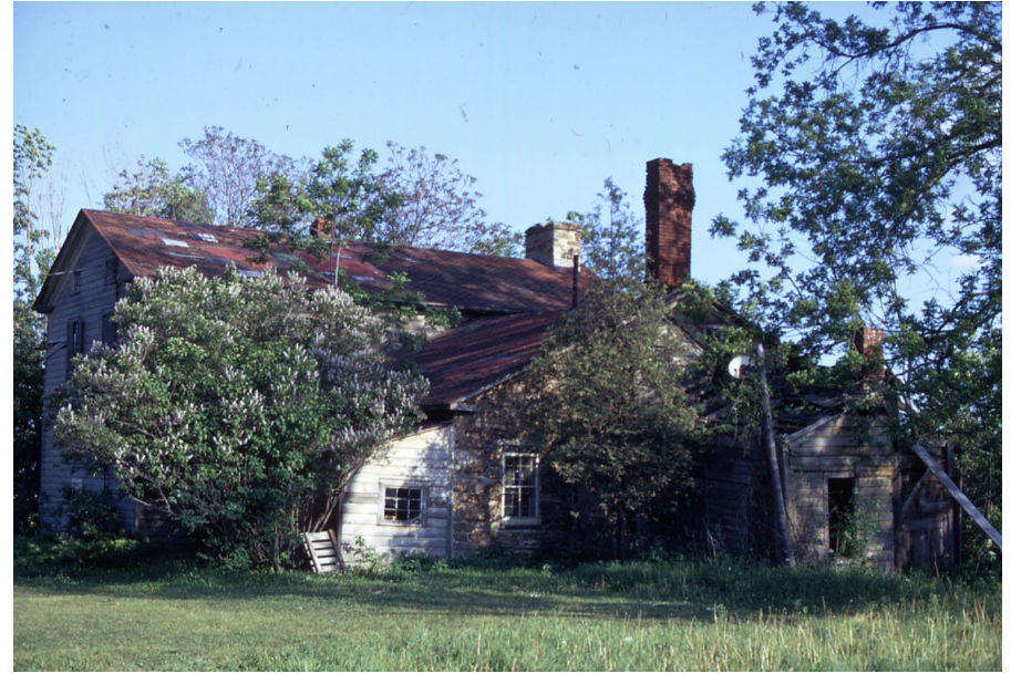
Fig. 11 Joseph De Rijck, "Cherry Hill House, Dixie," 1972, Mississauga Library System, I.D. MC0483. The corner view shows a reddish asphalt shingle roof over both the front part and stone back wing. Patches over the asphalt shingle are also evident.
