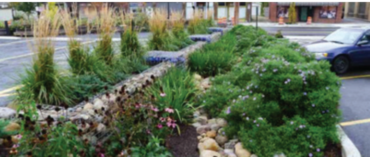
Post-construction bioretention implemented on private property in the Northeast Ohio Regional Sewer District, OH
