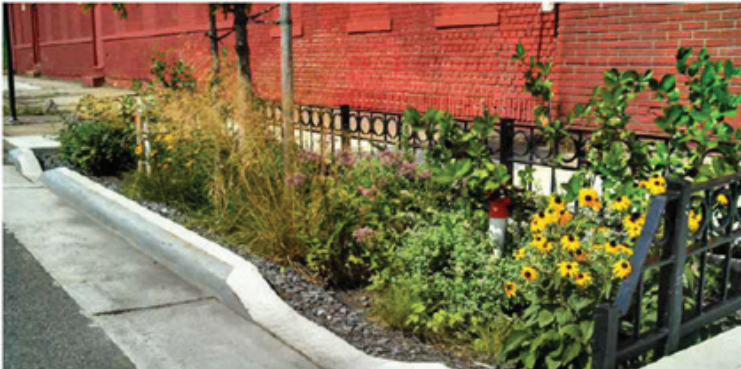
Right-of-way rain garden in New York City, NY
