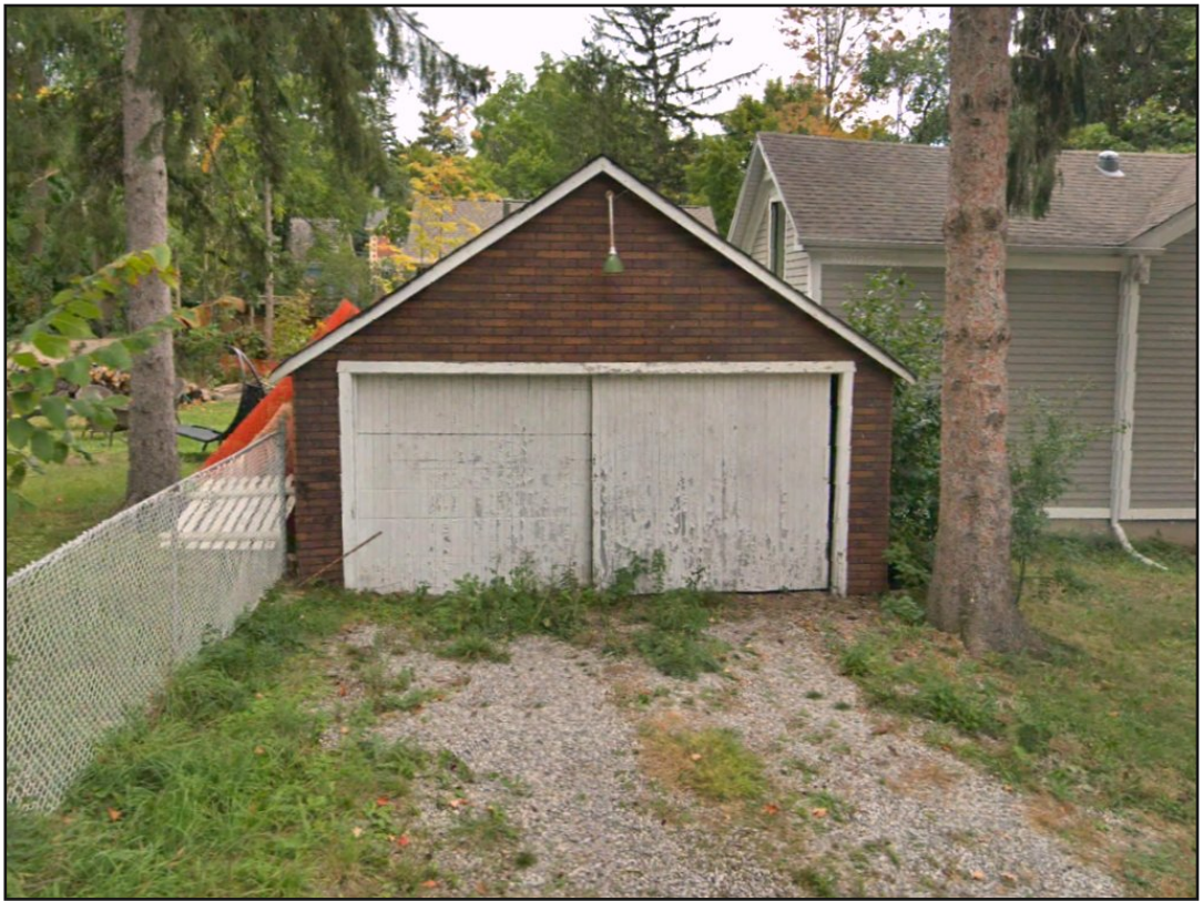
2.3.2c: front (north) elevation of garage
