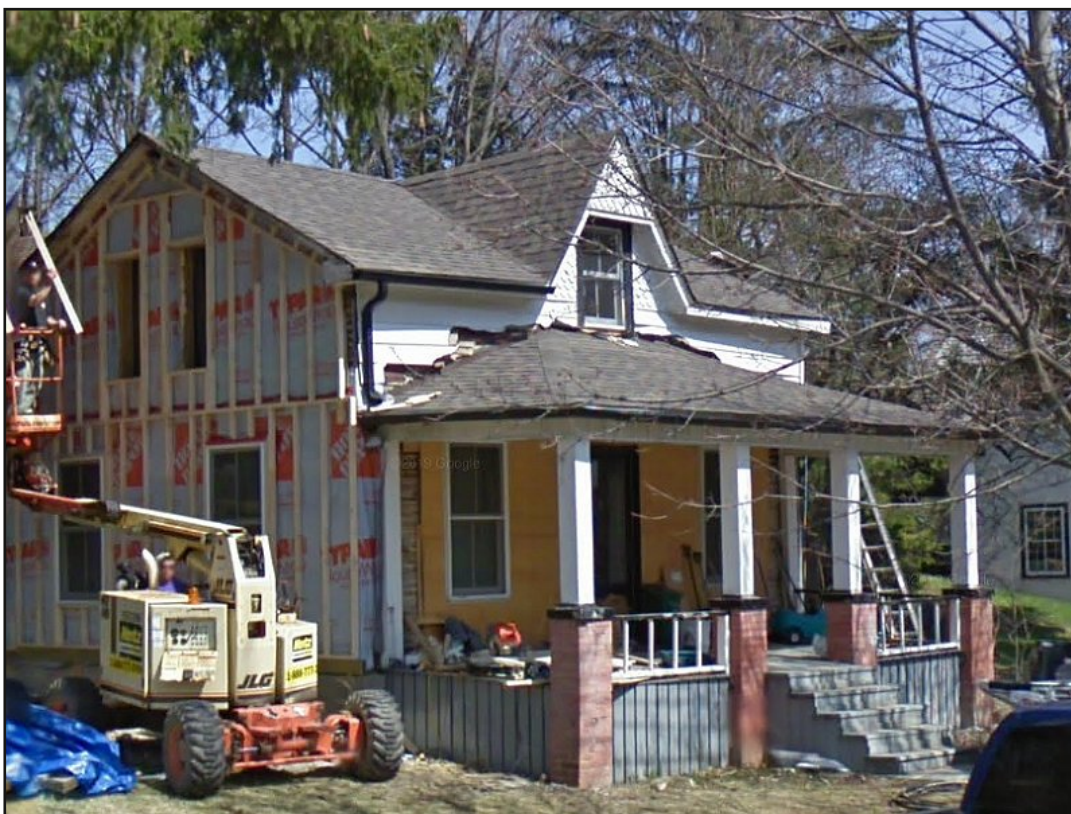
2.3.6d: 7025 Pond Street, main residence in April 2009
