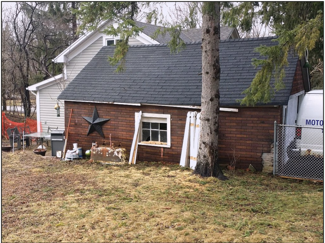
2.3.2g: east and north elevations of garage
