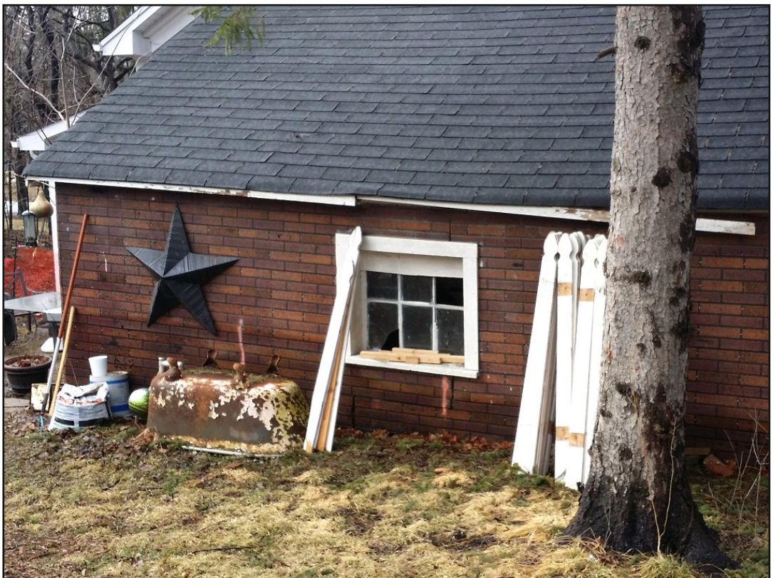
2.3.2h: east elevation of garage
