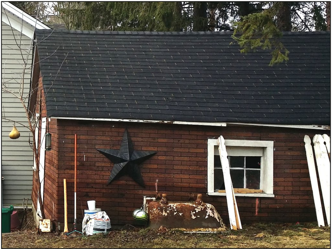
2.3.2e: east elevation of garage
