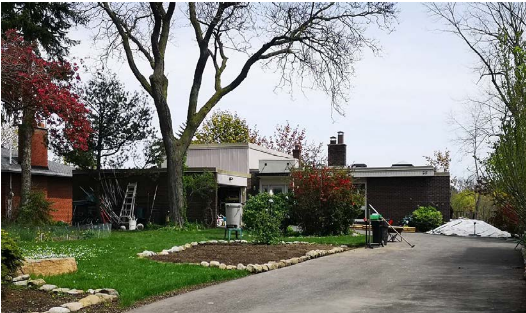
25 Plainsman Rd. This building is strongly similar to 11 Plainsman Rd.
