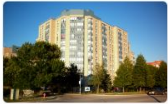
Net Zero Carbon Retrofit of an Affordable Housing Facility, Weaver's Hill
