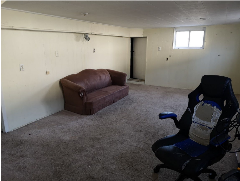
Basement Family/Recreation Room – note non-professional construction
