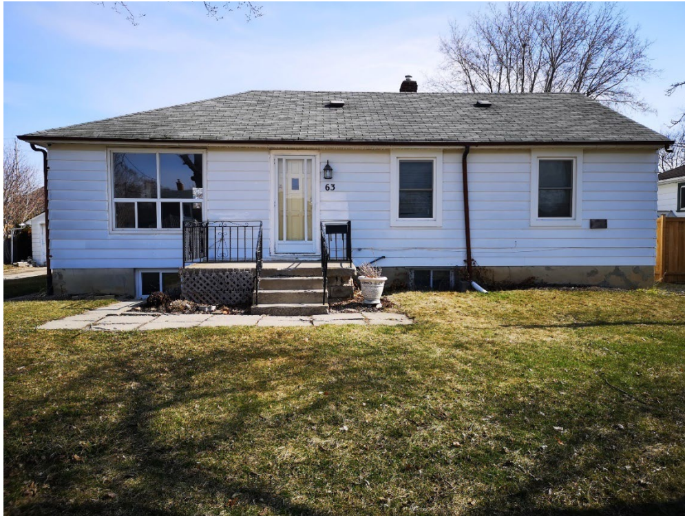
Front Elevation – note hipped roof on left, gable on right. Front porch was a later addition
