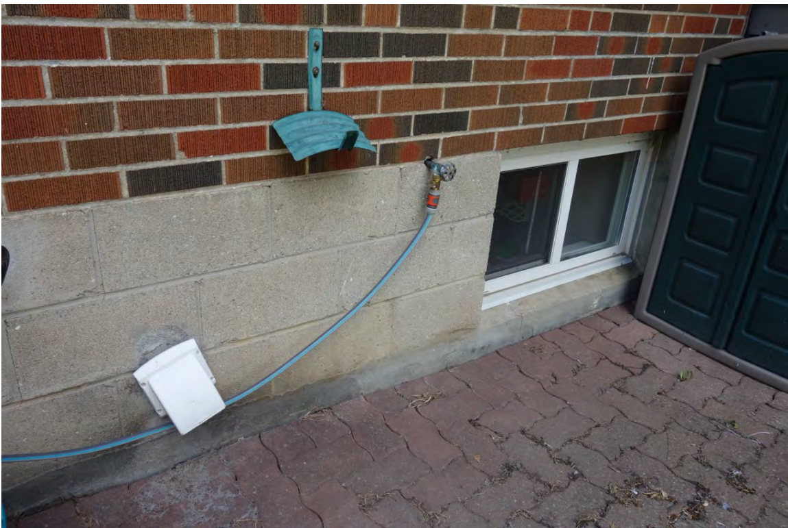
DETAIL – concrete block foundation
