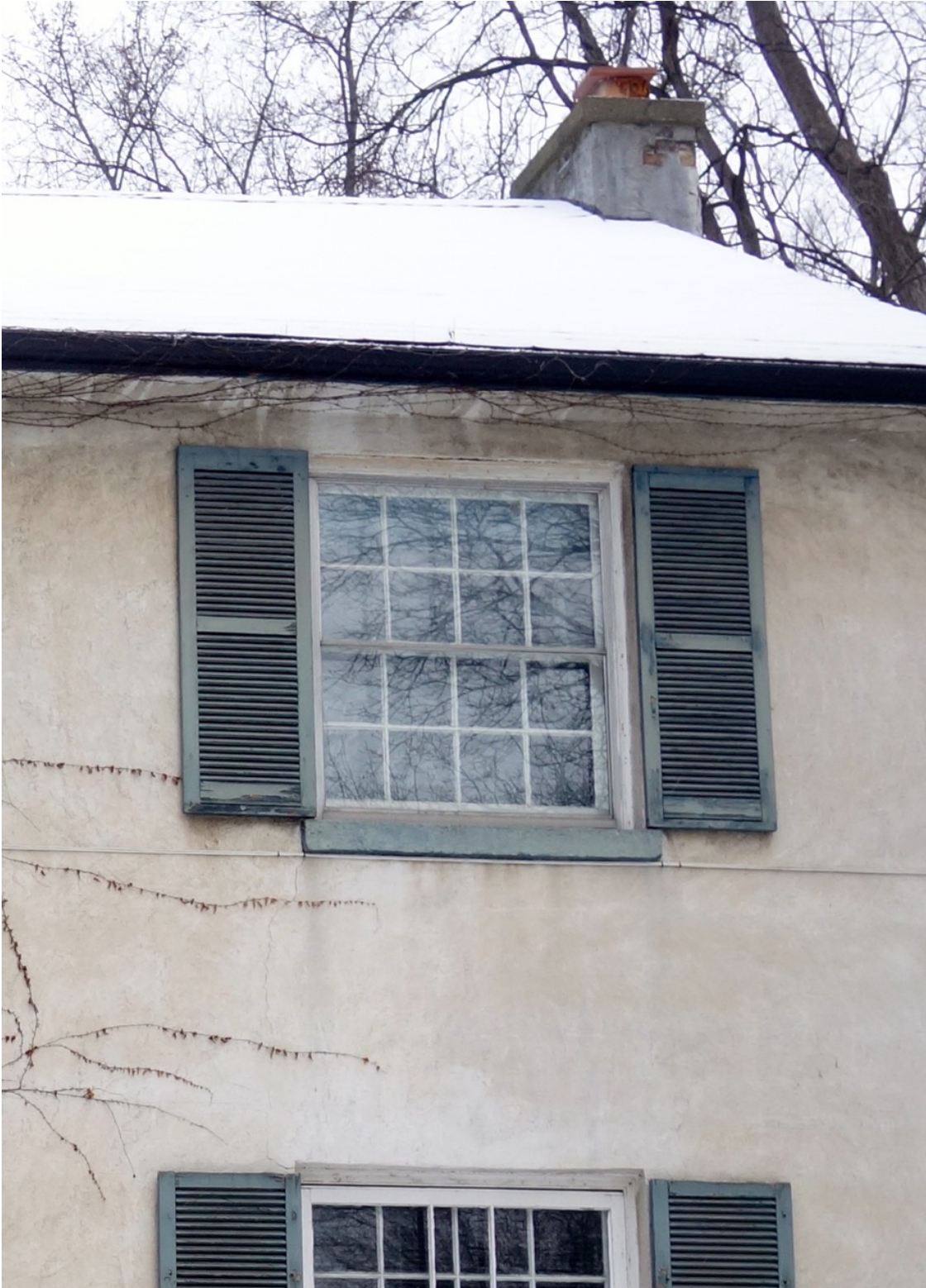
2 nd FLOOR WINDOW ON MAIN ELEVATION – 8 over 8 configuration - new putty, paint and some repairs needed on wood windows and shutters
