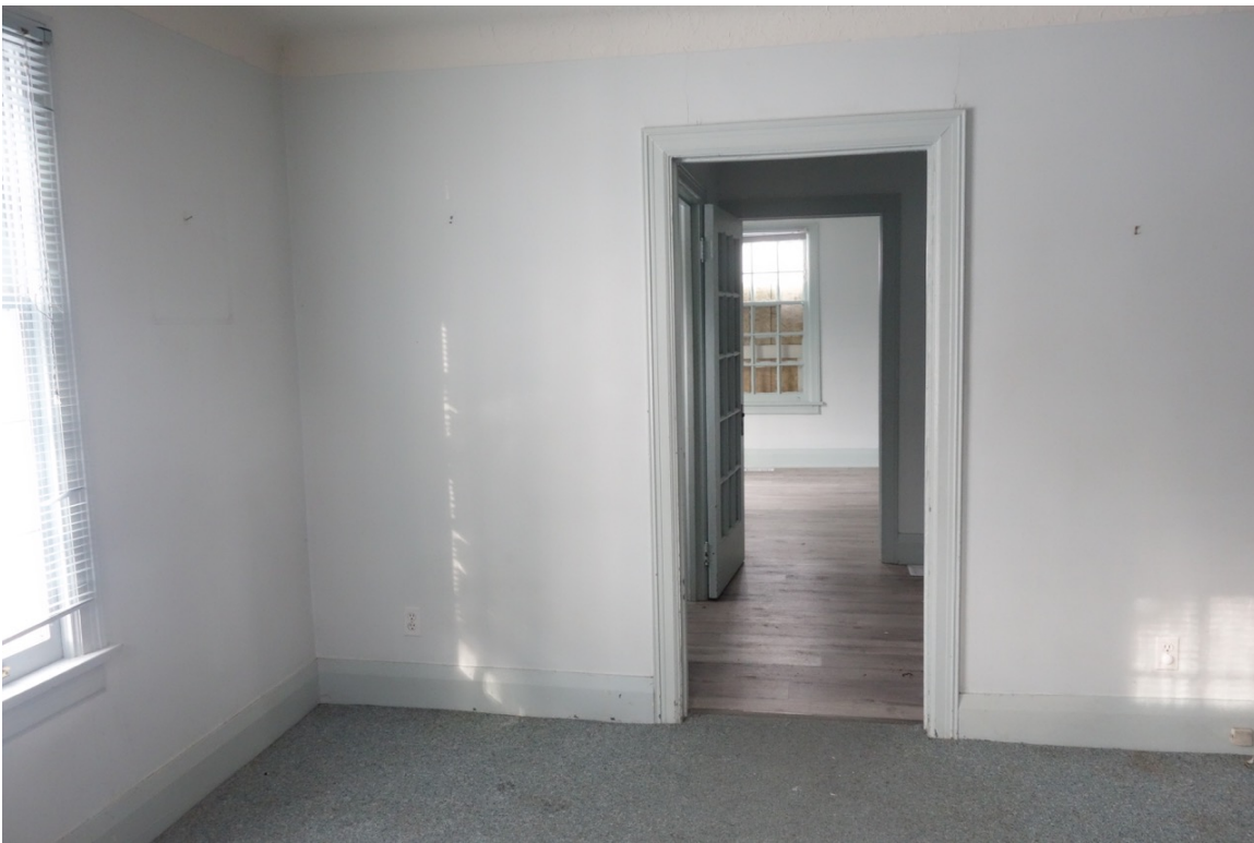
DINING ROOM – original baseboard, door and window casings
