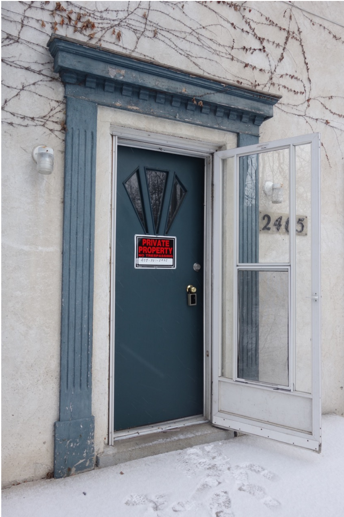
MAIN ENTRANCE – replacement door – exposed wood where paint finish has failed
