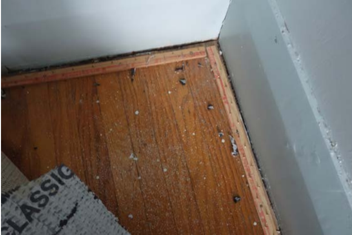
2 ND FLOOR HALL – original oak flooring well preserved beneath the wall-to-wall carpeting
