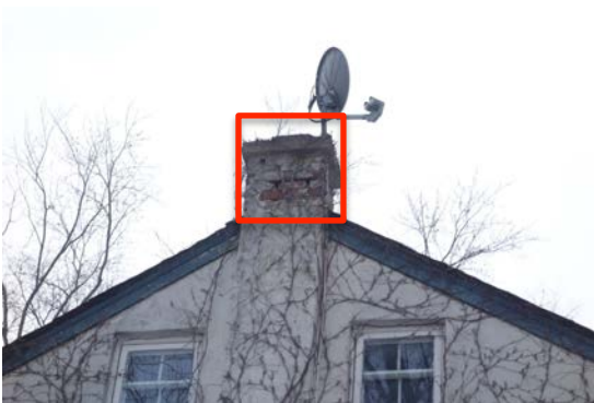
Original lime stucco has failed on the chimneys and is cracking in other areas
