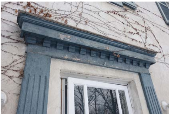
Original wood components are intact but have not been well maintained
