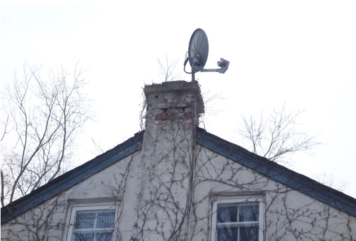
BRICK WITH STUCCO - chimney needs re-building and stucco repair
