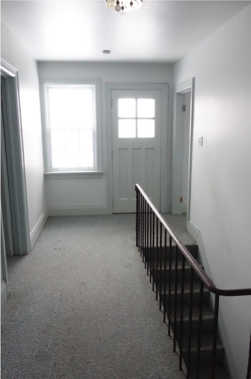
2 ND FLOOR HALL – replacement iron railing – original wood doors, baseboard and trim – modern wall-to-wall carpeting
