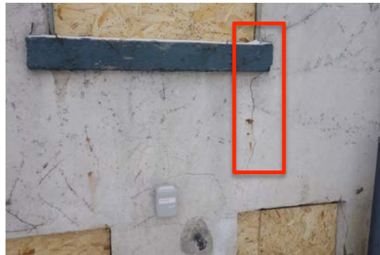
Original lime stucco has failed on the chimneys and is cracking in other areas
