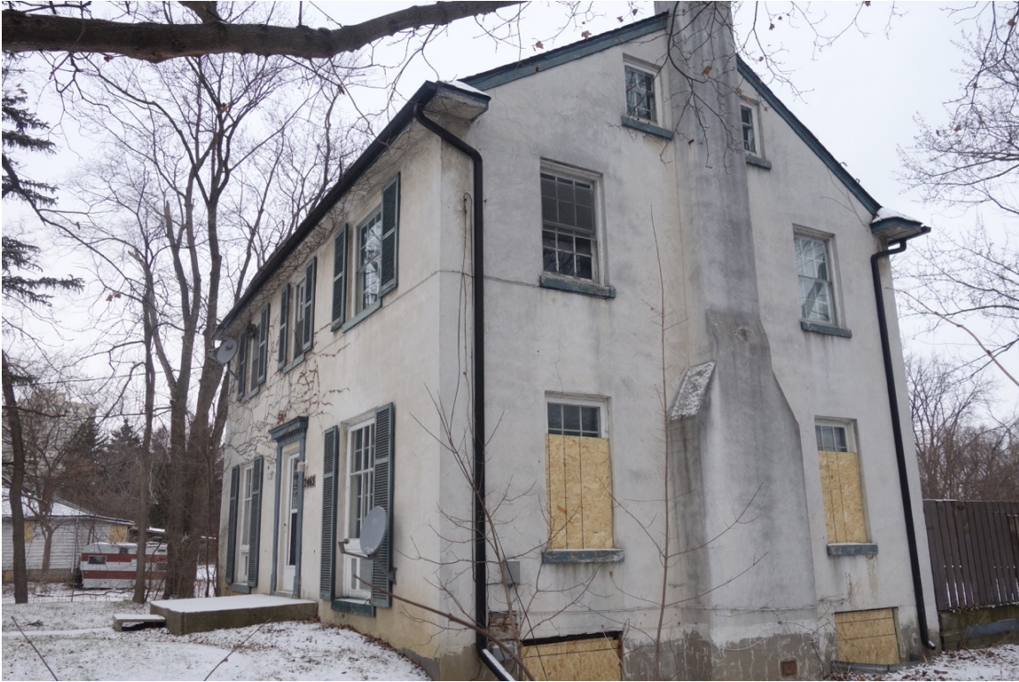
FRONT & SIDE ELEVATIONS – carbon deposits on wet area of the stucco
