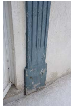
Original wood components are intact but have not been well maintained
