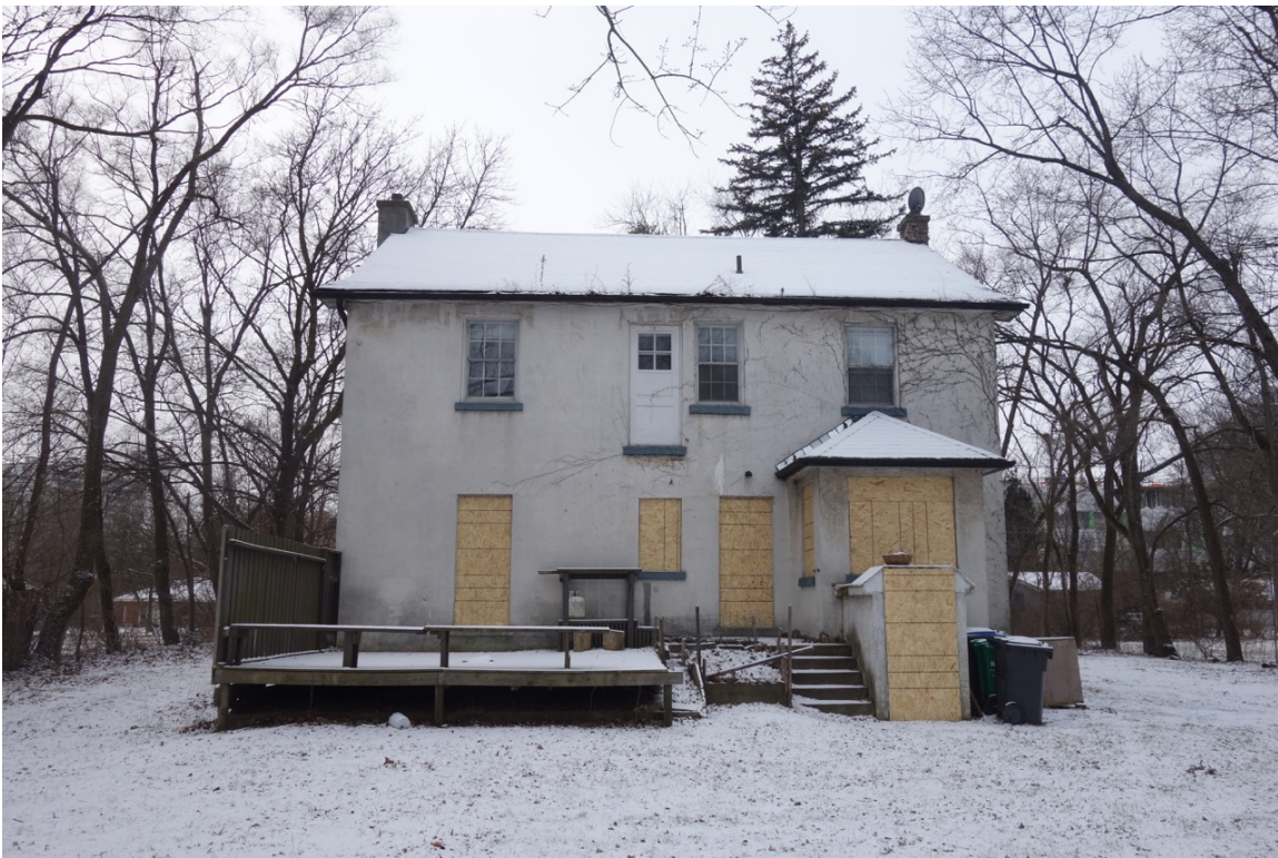
REAR ELEVATION – vegetation has grown up into the soffit and roof gutter
