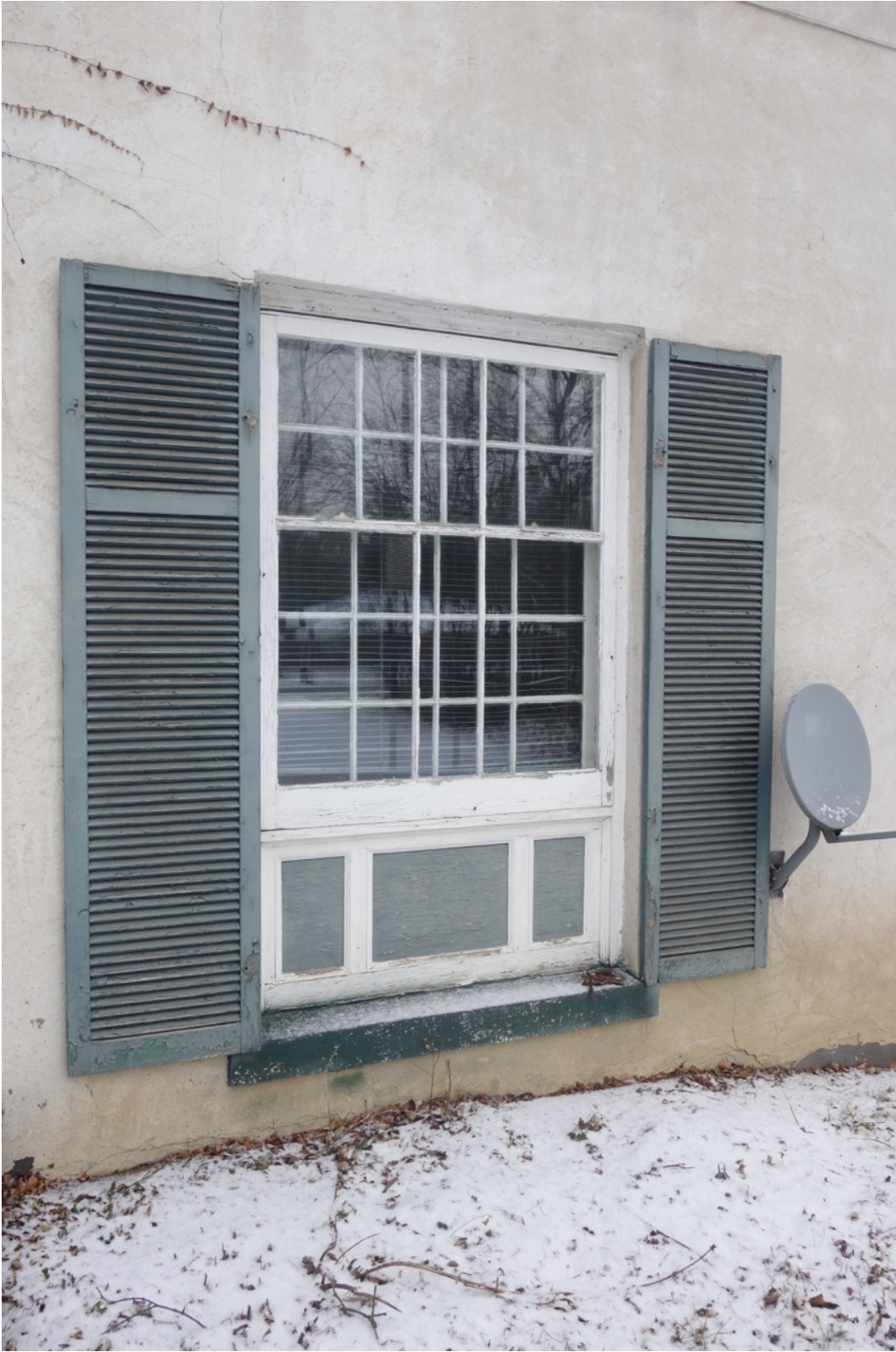
GROUND FLOOR WINDOW ON MAIN ELEVATION – 8 over 12 configuration - new putty, paint and some repairs needed on wood windows, shutters and paneling
