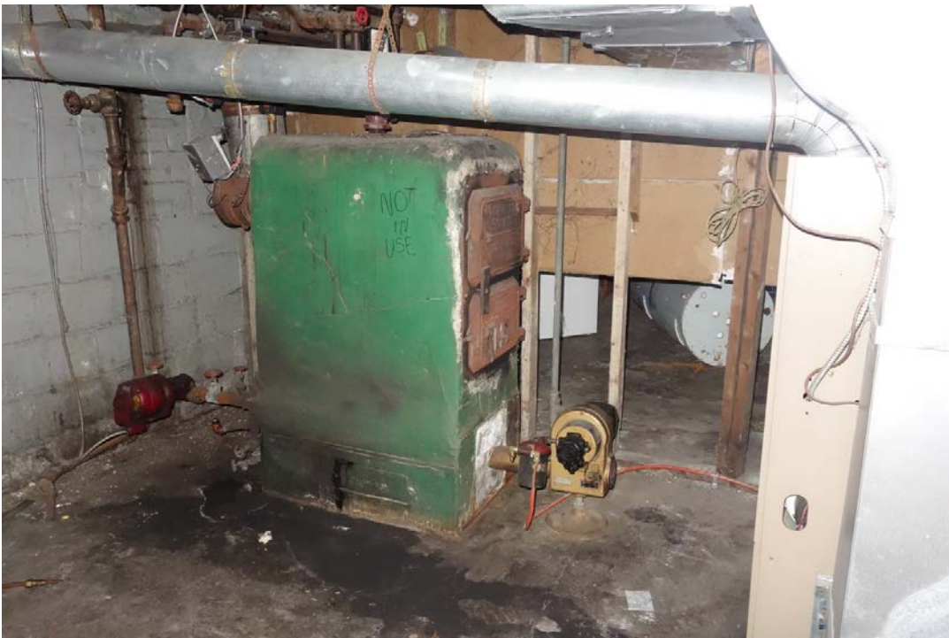
BASEMENT – original furnace
