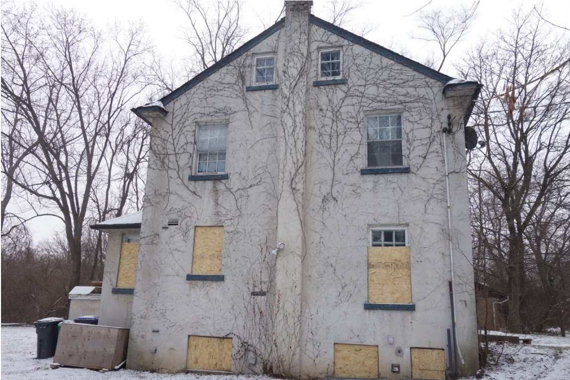
SIDE ELEVATION – ivy may have damaged stucco – missing downspout on left side - water staining below eaves and at grade level
