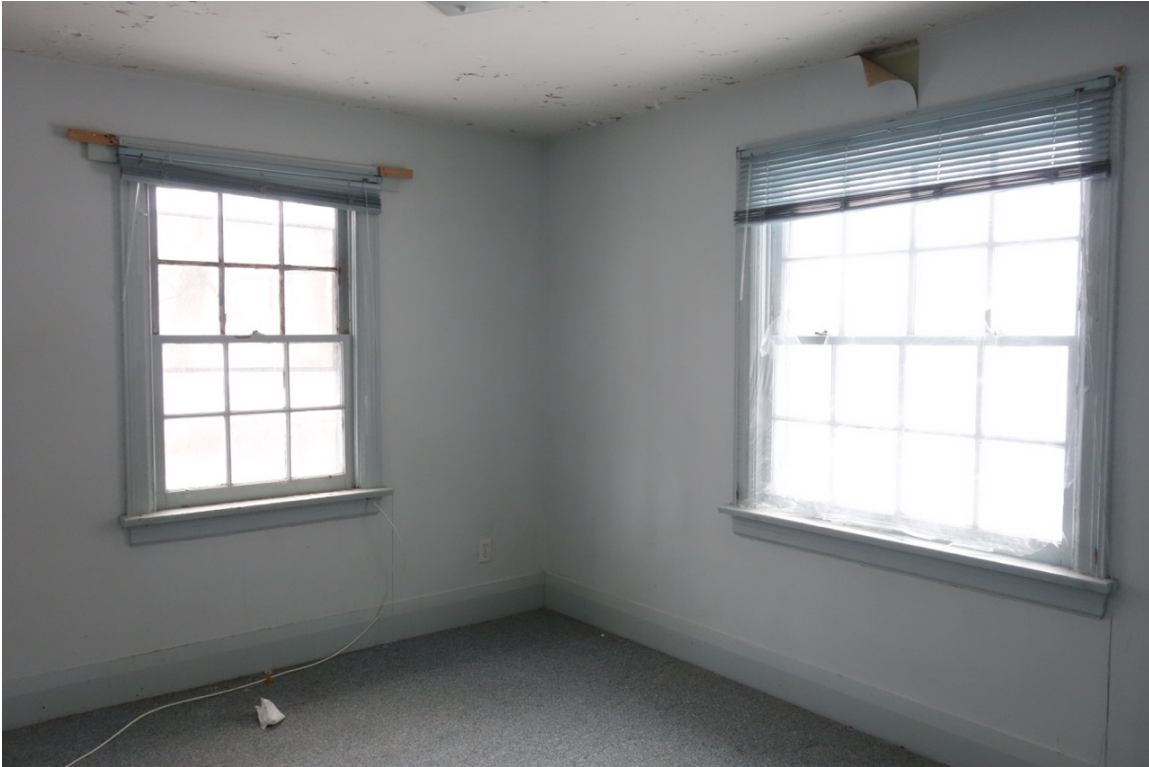
2 ND FLOOR - BEDROOM 2 – original windows – modern wall-to-wall carpeting – ceiling damage due to roof leaks
